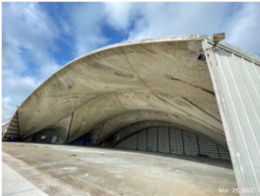
Photo 4: East G.A. Hangar No. 1 (Gault Hangar) hangar opening. Photo taken on the airport apron, facing southwest.
