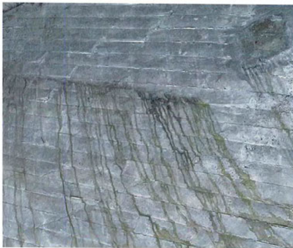
East GA Hangar No.1 Facing ceiling of Hangar.
