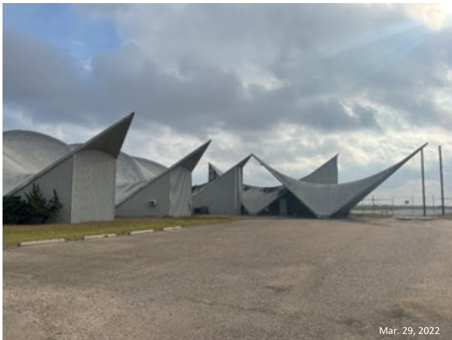
Photo 2: East G.A. Hangar No. 1 (Gault Hangar) main office/entrance and adjoining storage rooms. Photo taken on the south side of the building, facing east.
