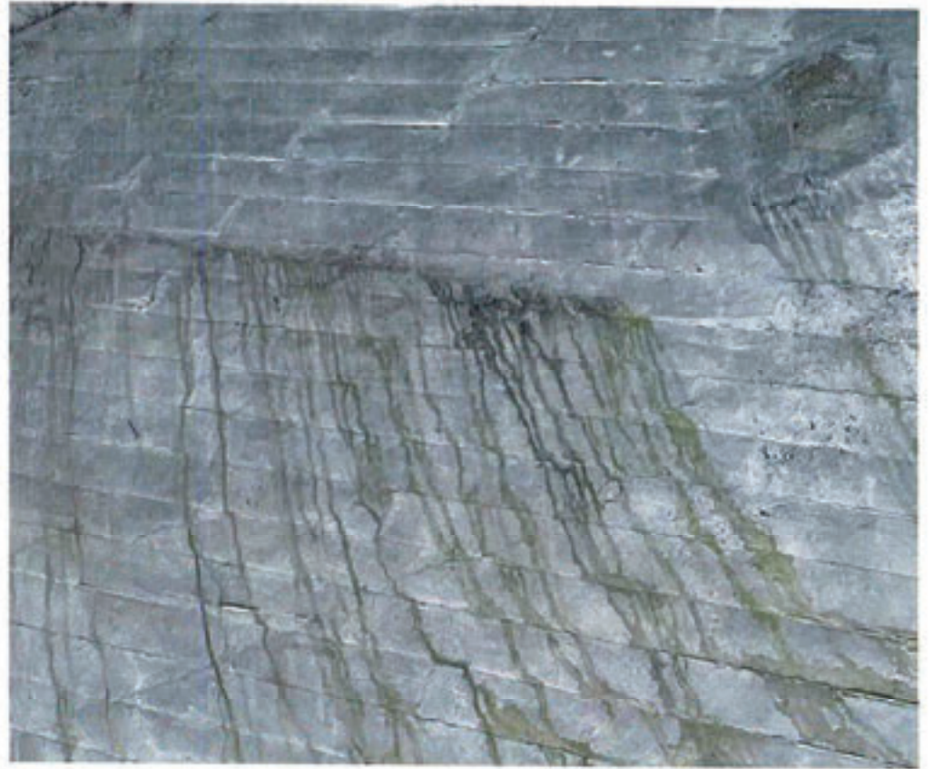
East GA Hangar No.1 Facing ceiling of Hangar.
