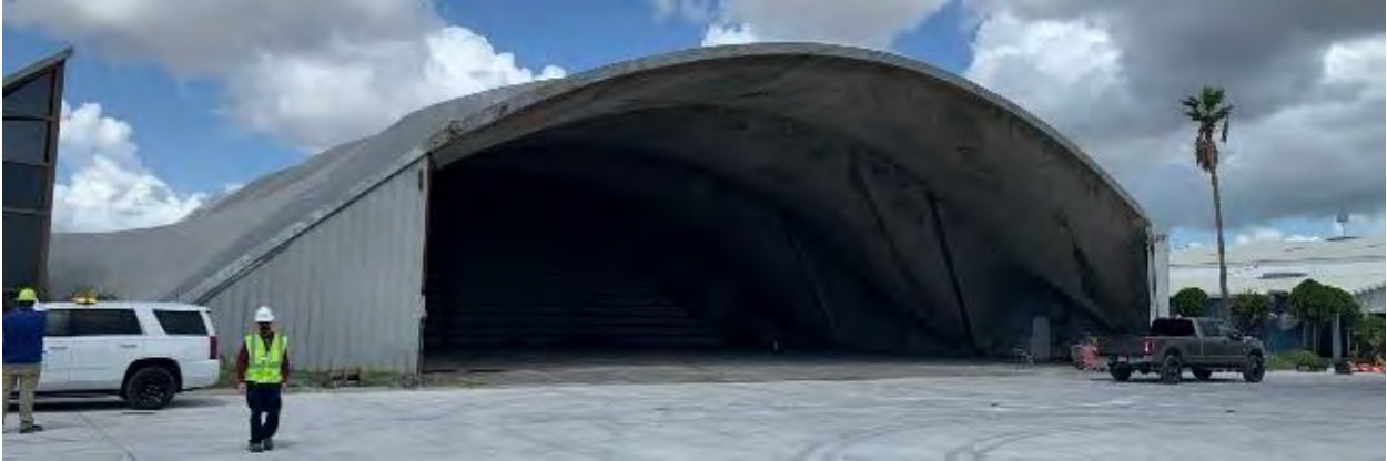
Photo 1. View of front side of Gault Hangar.
