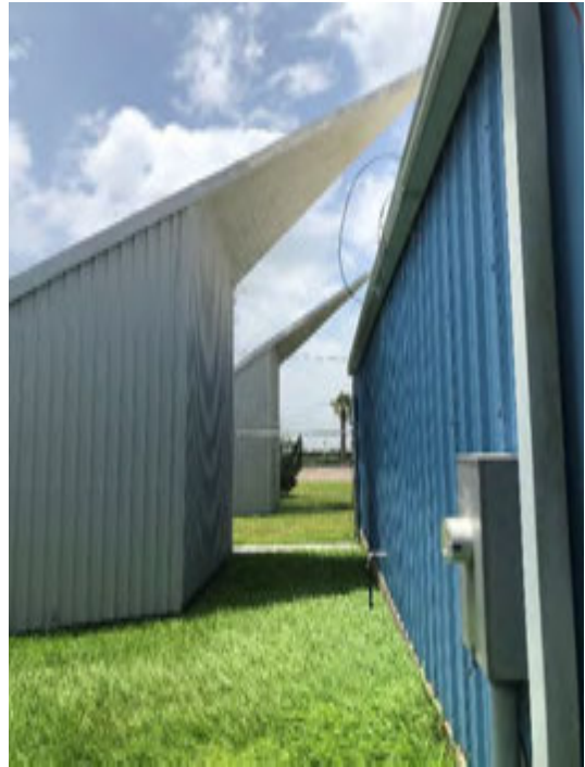
Photo 5. Concrete roof structure of Gault Hangar overhanging an adjacent office building.
