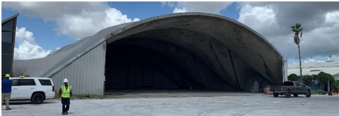
Figure 1: East G.A. Hangar No. 1 “Gault Hangar”
