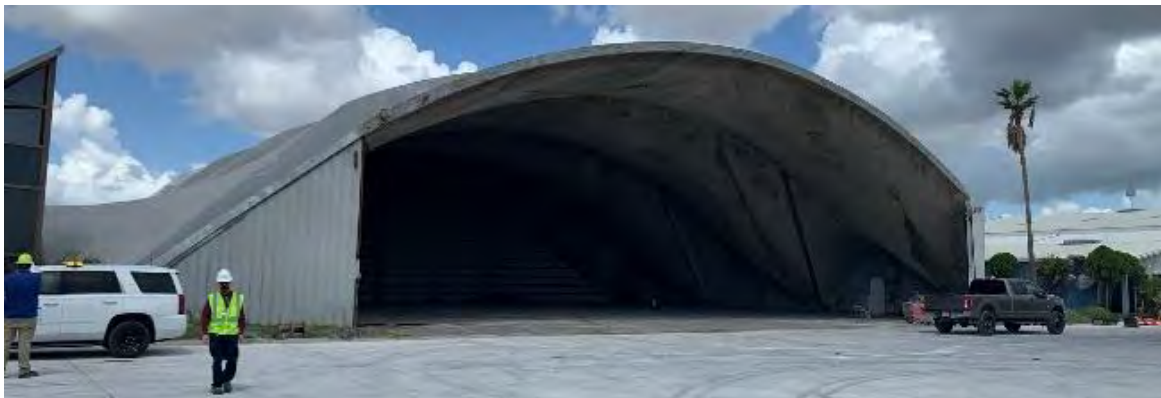
Figure 1: East G.A. Hangar No. 1 “Gault Hangar”
