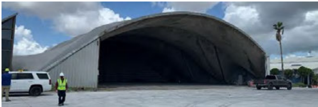
Figure 1: Existing EGA Hangar 1
