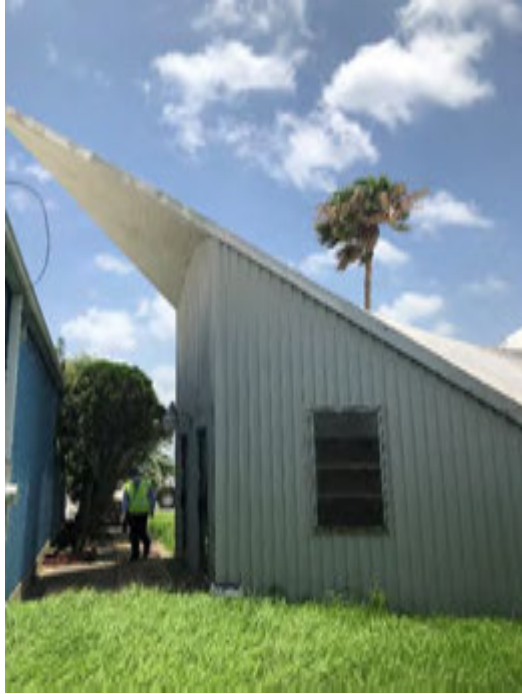
Photo 4. Concrete roof structure of Gault Hangar overhanging an adjacent office building.
