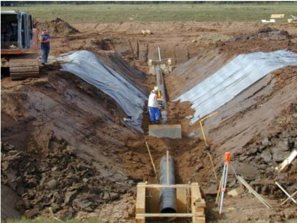
Figure 6. Culvert being replaced with high-density polyethylene pipe (Source: H. Kolstee, NSDAF, 2004)
