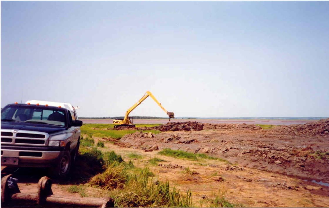
Figure 5. Construction of modern dyke (Source: H. Kolstee, NSDAF, 2004)
