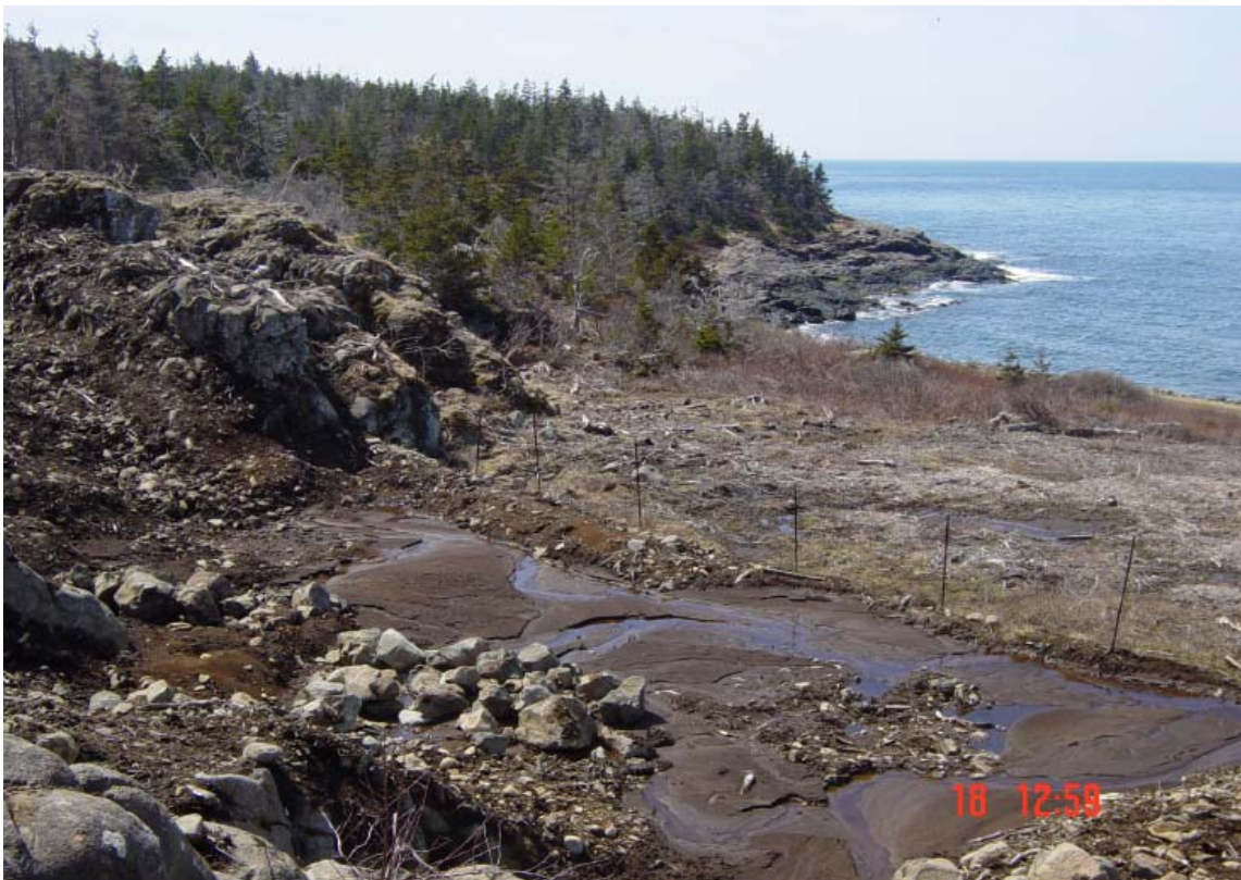
Figure 5. Sediment runoff from stripped hills on a proposed quarry site near the Bay of Fundy
