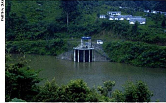
The entrance of the tunnel carrying water from the Ranganadi dam reservoir to the powerhouse at Hoz, 15 km from Yazali
