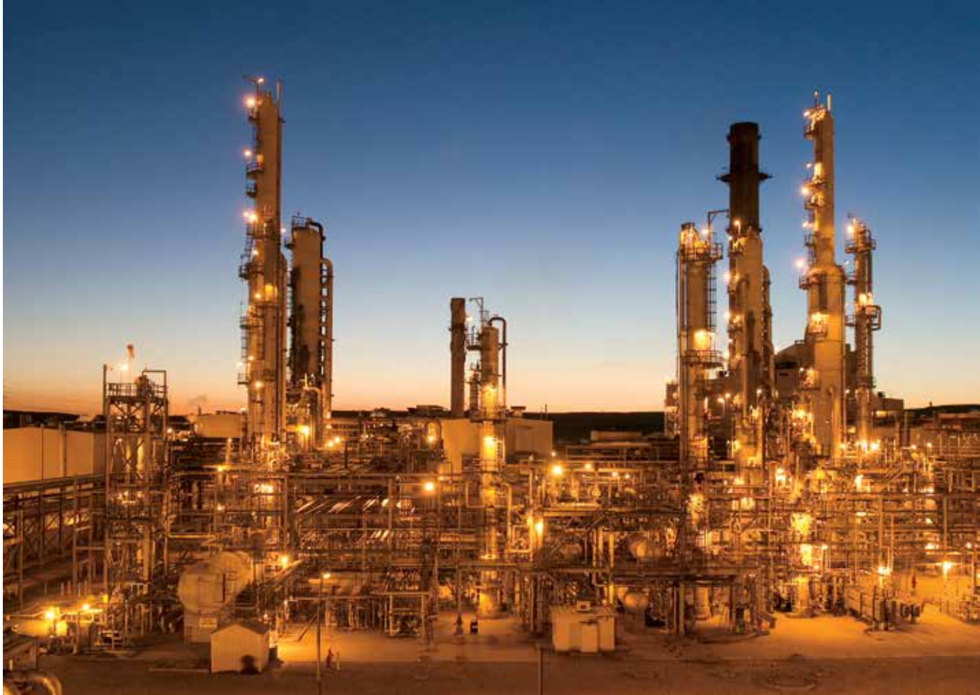
A portion of the Rectisol gas processing unit at the Great Plains Synfuels Plant at dusk. The Rectisol unit uses a cold methanol wash to separate the waste gas stream from the synthetic gas stream.
