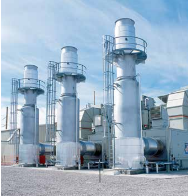
Barber Creek, 20 miles west of Gillette, WY, is one of three Basin Electric combustion turbine generator sites in northeastern Wyoming; the other two are Arvada and Hartzog. Each site consists of three generators, each with a generating capacity of five megawatts.
