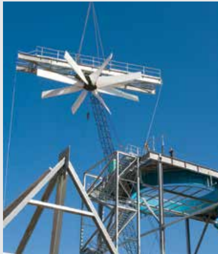
Top: Aerial view of the structural steel in place at Dry Fork Station on March 2009. Left: The first of 45 fan placements in September 2008 in the air-cooled condenser, where steam is condensed into water and recycled to the boiler. Right: Lift of the 240-ton steam drum into place on March 22, 2009. The steam drum, the heart of the boiler, is the first place where steam is collected before heading to the turbine and generator to make electricity.
