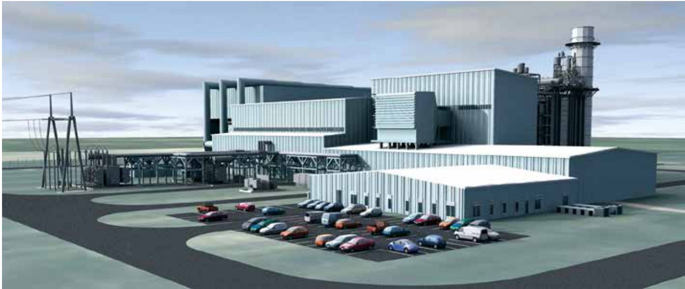
This is a site simulation of the 300-net-megawatt Deer Creek Station under construction near Elkton, SD, in Brookings County. Construction began on the combined-cycle station on July 27, 2010. The plant features two turbine-generator sets: one fired by natural gas; the other is driven by steam. Both of the turbines are connected to generators. The station is expected to be completed in 2012.
