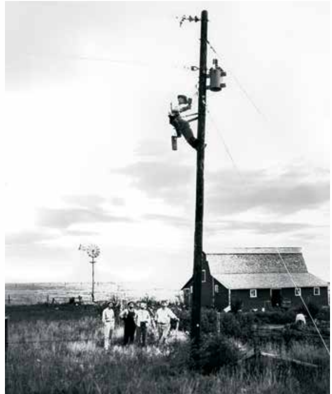
Lawrence Hughes, Williams Electric Cooperative superintendent, checks transformer output on the Nasner farm, northwest of Williston, ND. This was the first farm to receive REA current from this cooperative, according to the Williston Herald of Sept. 4, 1947. Williston State College Foundation, William E. (Bill) Shemorry Photograph Collection.
