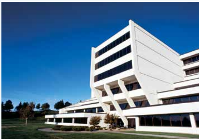
Basin Electric Headquarters
