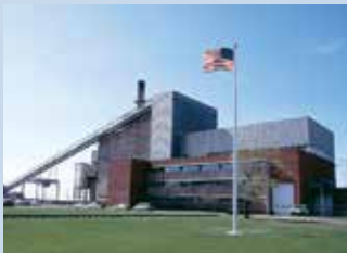
Earl F. Wisdom Station Unit 1 Owned and operated by Corn Belt Location: Spencer, IA Capacity: 38 MW winter, 37.5 MW summer Fuel: Coal Operational: 1960
