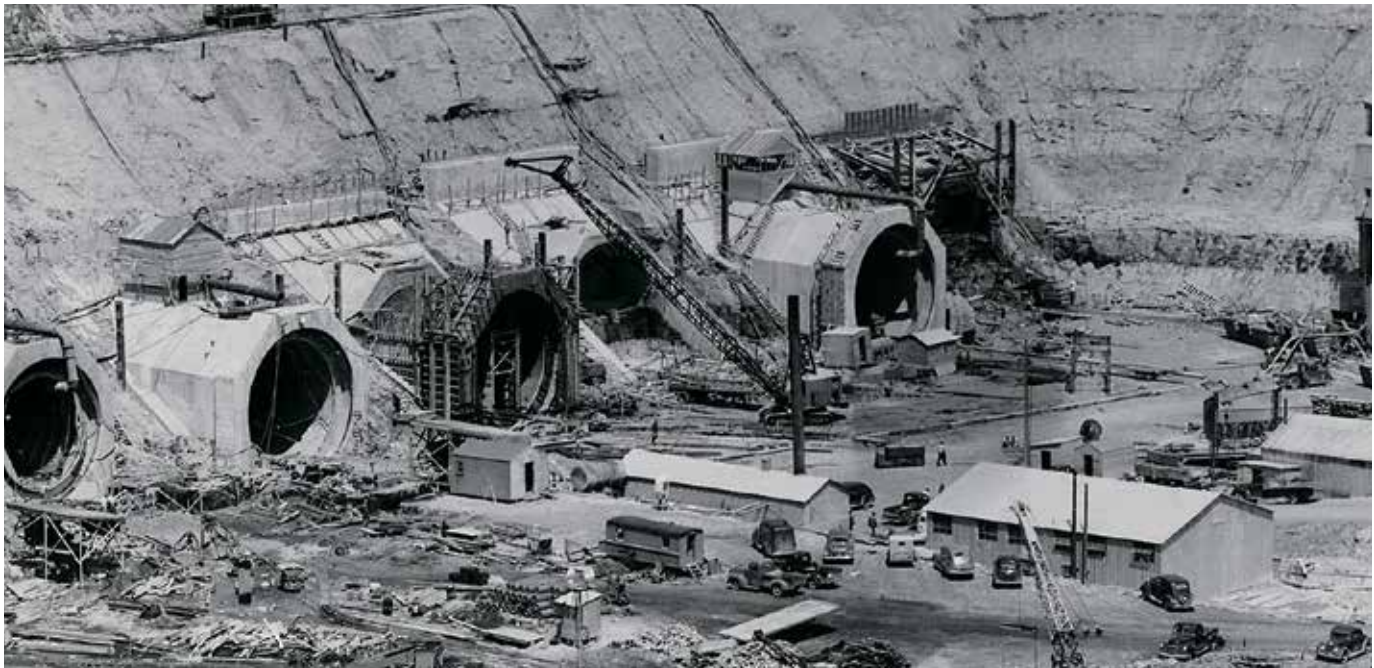
Construction of Garrison Dam in North Dakota took place from 1947-1954 at a cost of $300 million. The dam is 210 feet high and two-and-a-half miles long. Its embankment consists of 66.5 million yards of rolled earth fill.
