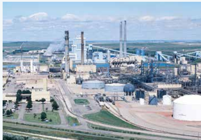
Great Plains Synfuels Plant
