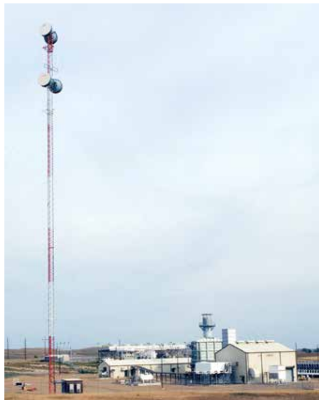
Basin Electric receives baseload generation from eight recovered energy generation units along the Northern Border Pipeline that use hot exhaust gas from compressor stations to produce electricity. This one is located near St. Anthony, ND.
