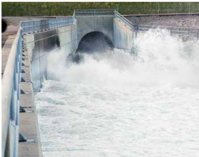
With a few years of higher-than-normal precipitation, the Missouri River system was flush with water. Water was discharged through the Oahe Reservoir's outlet tunnels in September 2010.
