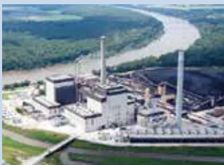
Walter Scott, Jr. Energy Center units 3 and 4 Operated by MidAmerican Energy Location: Council Bluffs, IA Capacity: Unit 3, 690 MW; Unit 4, 800 MW (Corn Belt's share, Unit 3, 26 MW; Unit 4, 42 MW) Fuel: Coal Operational: 1978 and 2007
