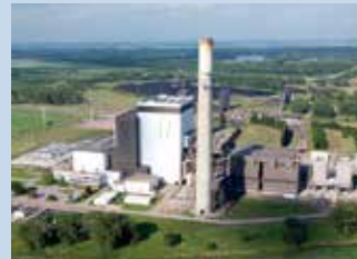
George Neal Station Unit 4* Operated by MidAmerican Energy Location: Sioux City, IA Capacity: 644 MW (Corn Belt Power's share, 75 MW) Fuel: Coal Operational: 1979
