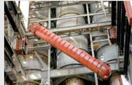
Top: Aerial view of the structural steel in place at Dry Fork Station on March 2009. Left: The first of 45 fan placements in September 2008 in the air-cooled condenser, where steam is condensed into water and recycled to the boiler. Right: Lift of the 240-ton steam drum into place on March 22, 2009. The steam drum, the heart of the boiler, is the first place where steam is collected before heading to the turbine and generator to make electricity.
