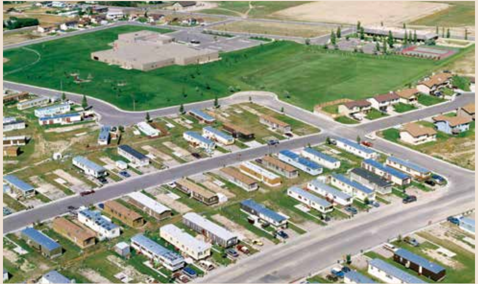
Black Mountain Village, a 185-acre subdivision, consisted of about 1,000 housing units including mobile homes, campers, “bachelor” quarters, single family houses, and a recreation center, cafeteria, and shower and laundry facilities.
