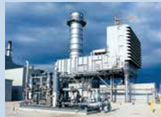
Earl F. Wisdom Station Unit 2** Operated by Corn Belt, 50% ownership Location: Spencer, IA Capacity: 80 MW winter, 78.2 MW summer Fuel: Natural gas/fuel oil Operational: 2004
