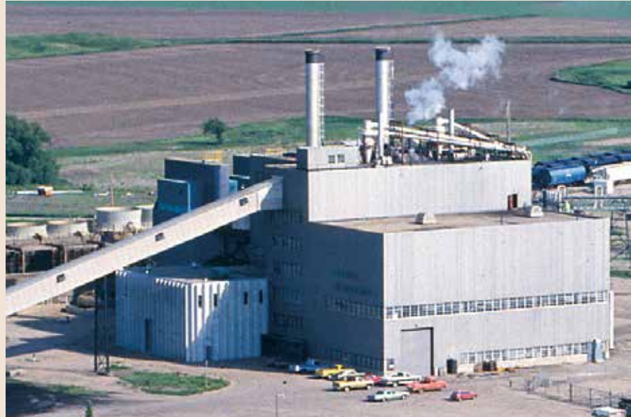
The William J. Neal Station as it appeared in the early 1980s. The plant no longer exists. It was dismantled in 1999.
