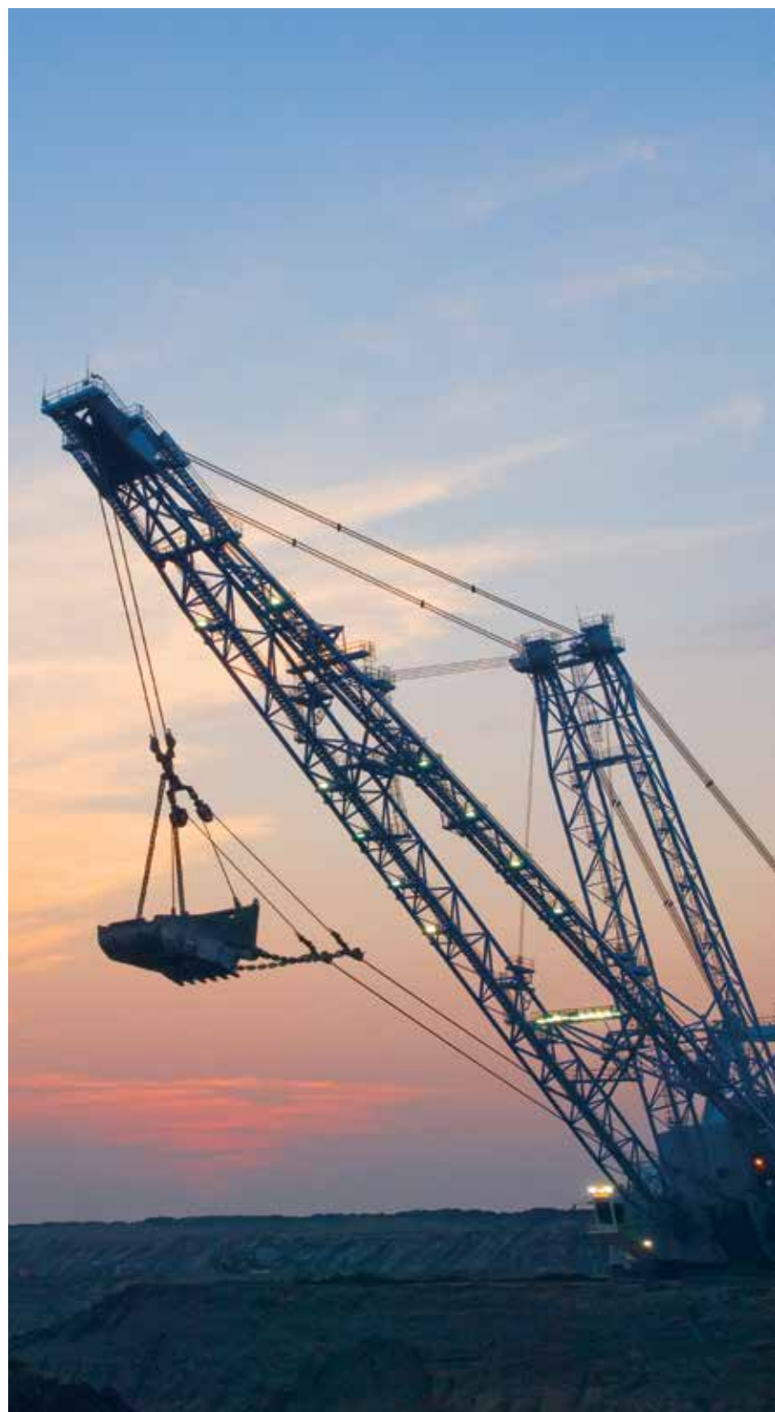
Two Freedom Mine draglines generally operate 24-hours a day, seven days a week to remove overburden from coal seams. They each weigh 13 million pounds and move 150 tons of earth per minute. The buckets hold 124 cubic yards of earth, which is equivalent to 2,770 bushels of wheat or a half million golf balls.
