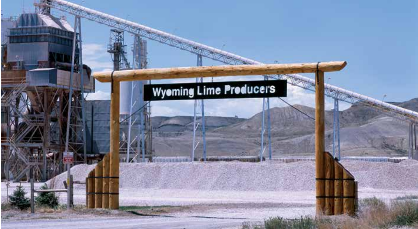
To help control costs of the Clean Air Act amendments, Basin Electric subsidiary, Dakota Coal, built a lime kiln. Lime is used for water treatment and in power plant scrubbers to remove sulfur dioxide emissions. The kiln is 1.5 miles north of Frannie, WY.
