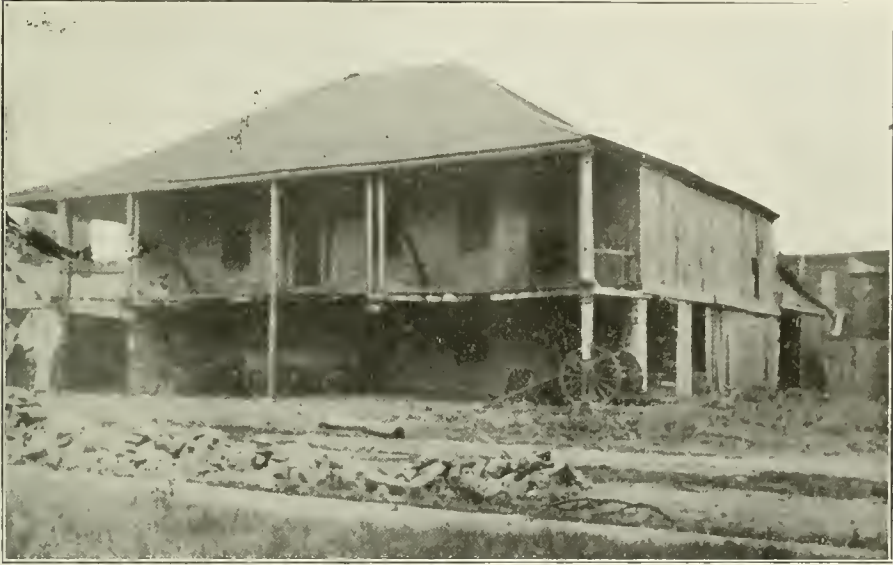
OLD GOVERNMENT BUILDING, FORT SCOTT
