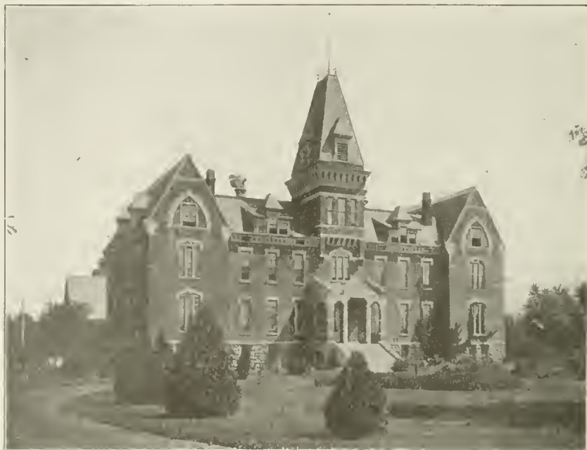
MAIN BUILDING, BOYS' INDUSTRIAL SCHOOL.
