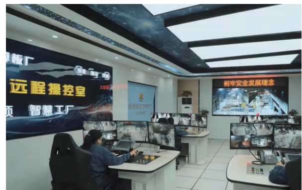
Huawei working with China Mobile Hunan to help Valin Xiangtan Iron & Steel, a factory in China's Hunan Province, use 5G to remotely control its cranes
