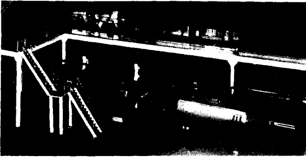
Fig. 1 Model of new "Gelsenkirchen" (Germany) 17,250-kw heat-power CCGT plant under construction. Cycle data: Inlet pressure = 38 kg/sq cm; inlet temperature = 720 C; Fuel: blast-furnace gas and oil; Heat production = 17 \times 10^6 kcal 68.10^6 Btu/h). In foreground: Precooler and intercoolers for hot-water production. Recuperator below turbine group
