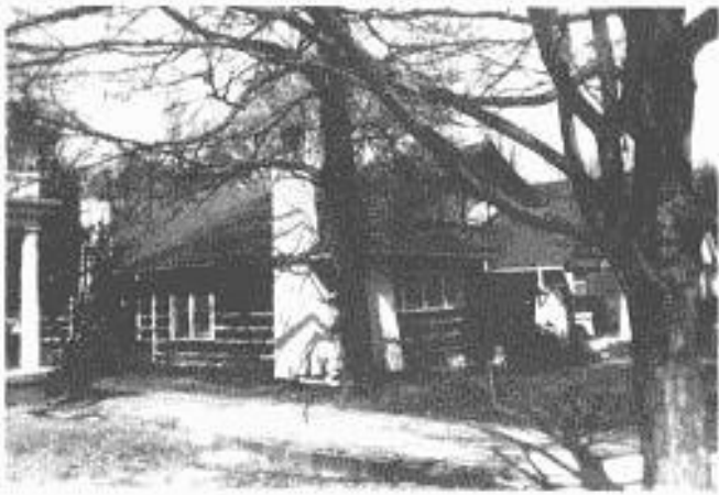
Figure 5. Southeast view of Clark Woodard's log bungalow, no visible foundation material noticeable.
