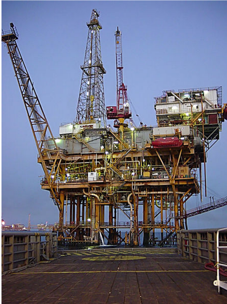
Figure 14.26: Oil platforms like this one of the coast of the Gulf of Mexico can be fixed or they can float. They are generally used on the continental shelf but new technology allows them to be in deeper places. (5)
