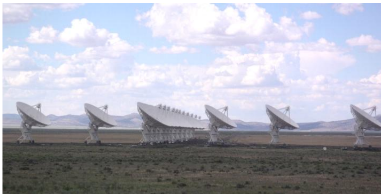
Figure 23.10: The Very Large Array in New Mexico has 27 radio dishes, each 25 meters in diameter. When all the dishes are spread out and pointed at the same object, they act like a single telescope with a diameter of 22.3 mi. (7)
