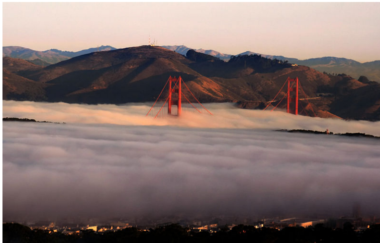
Figure 16.9: Advection fog fills the gap where the Golden Gate Bridge spans the San Francisco Bay inlet. (16)
