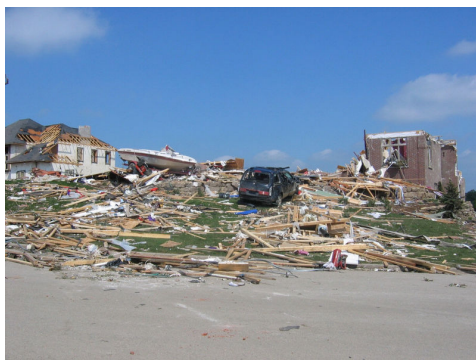
Figure 16.28: Tornado damage at Stoughton, Wisconsin in 2005. (41)
