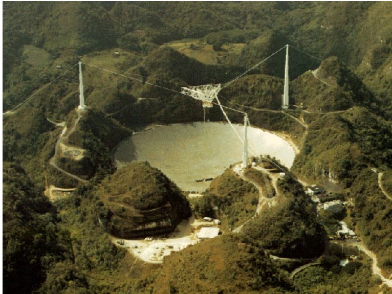
Figure 23.9: The radio telescope at the Arecibo Observatory in Puerto Rico has a diameter of 305 m. (1)
