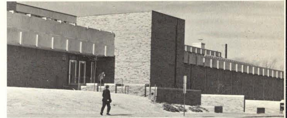
The CAC building is one of the busiest places on campus.
