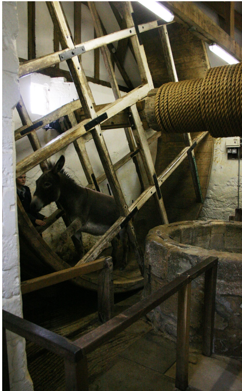
Figure 30 A donkey wheel operated well at Carisbrooke Castle
