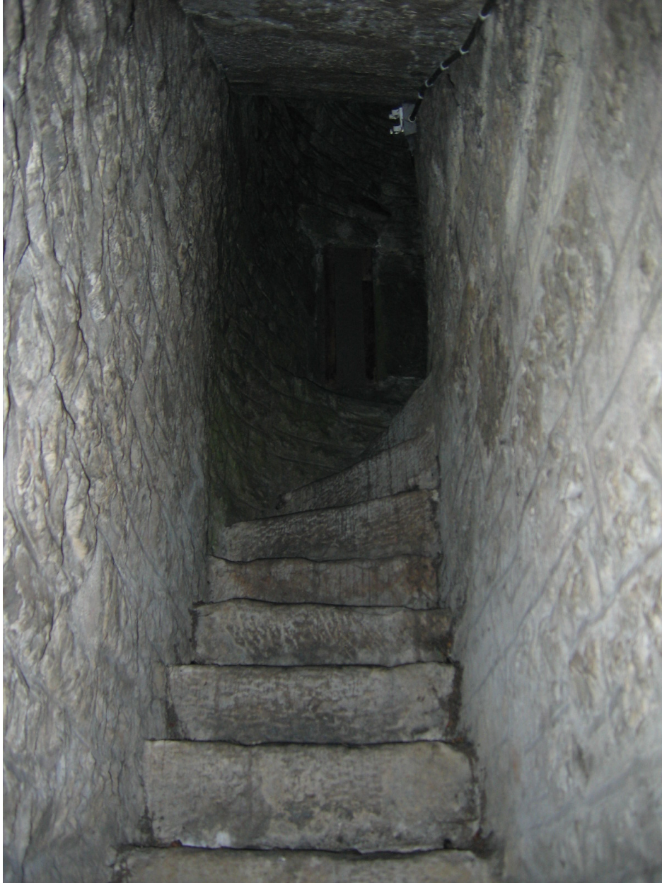
Figure 29 A typical castle staircase in turnpike design, this one is at Foulksrath Castle
