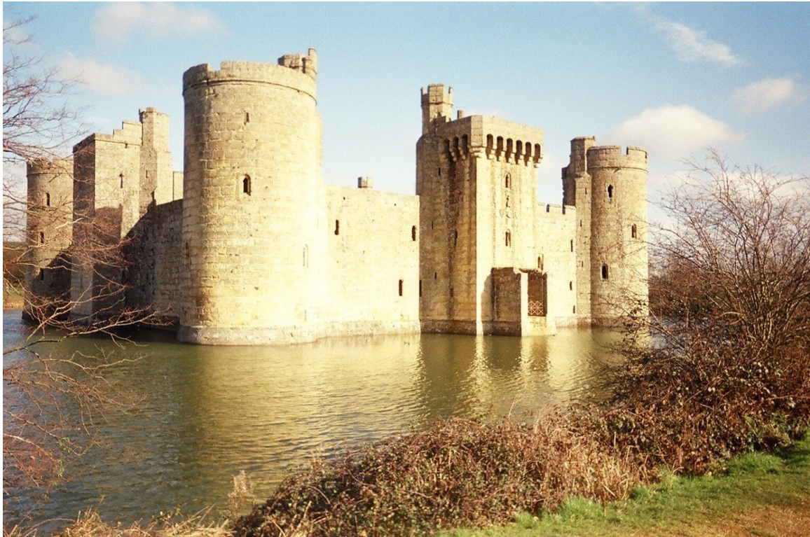
Figure 20 Bodiam Castle showing the extensive moat protecting the walls
