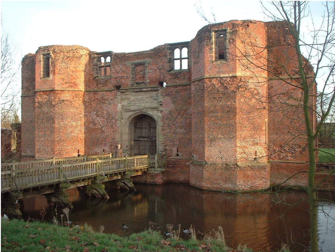
Figure 14 Kirby Muxloe Castle, a fine example of a brick built castle
