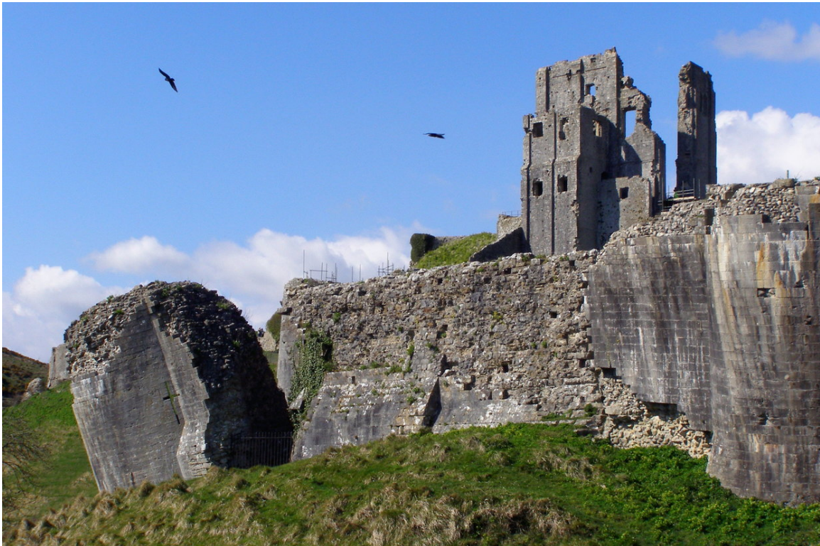
Figure 15 Corfe Castle in Dorset. In the foreground is the bailey wall, which was deliberately destroyed ("slighted") following the Civil War in order to render the defences useless
