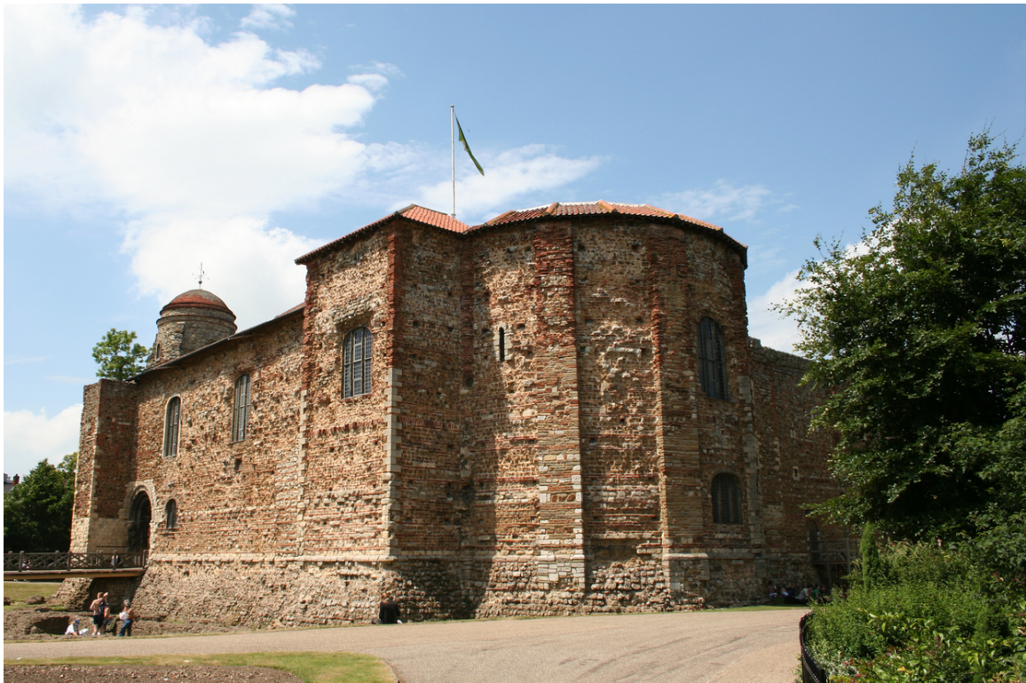
Figure 5 Colchester Castle in Essex. It was constructed from bricks recycled from Roman fortifications
