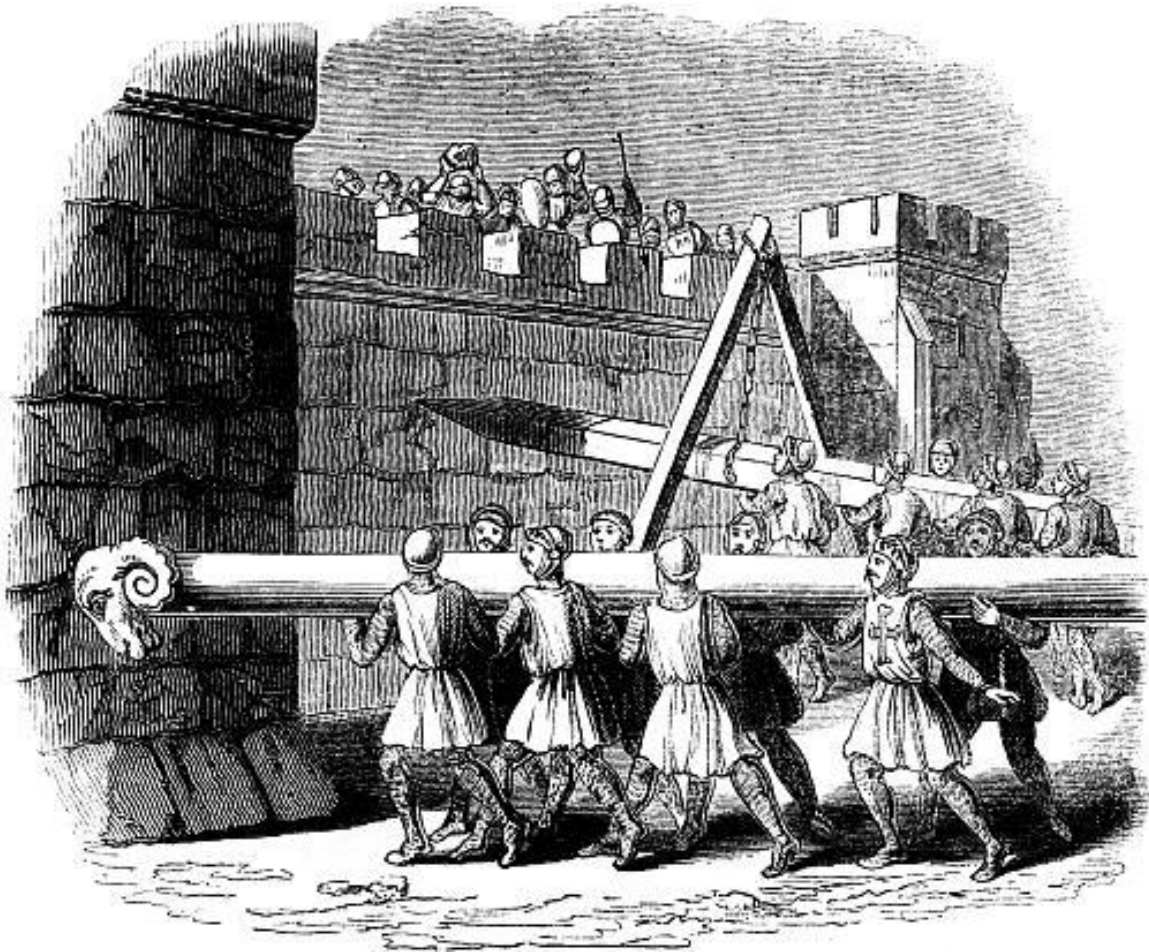
Figure 37 Attack on the walls of a besieged town with a battering ram.
