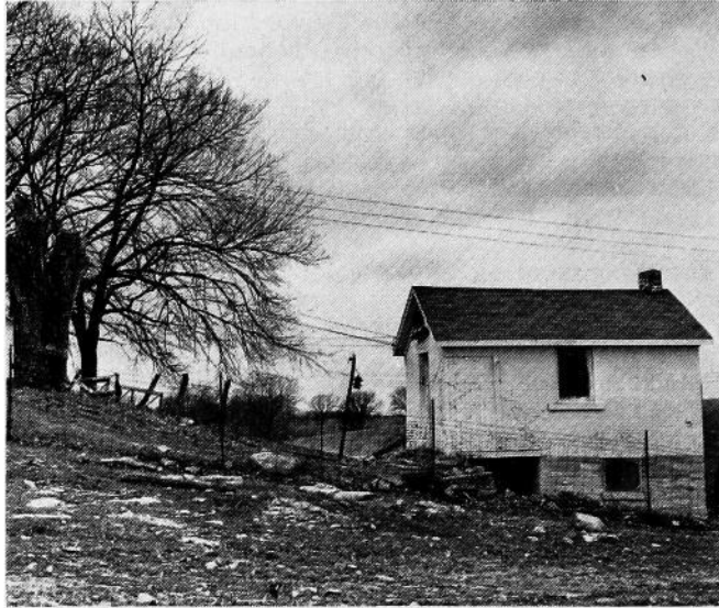
Old Spring house at Camp Harlan. Soldiers' initials whittled in its stone walls are plainly visible.
