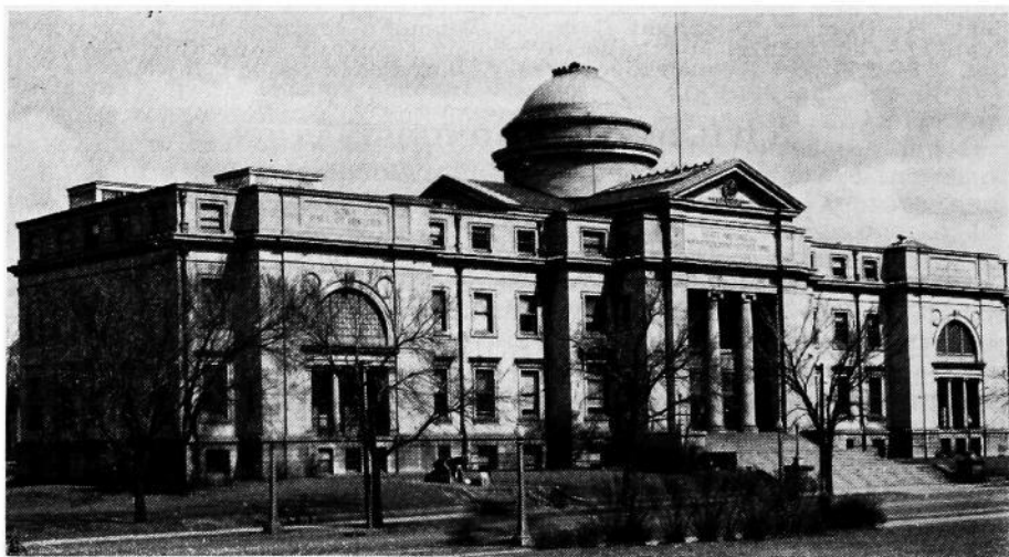
Historical Building, Des Moines
