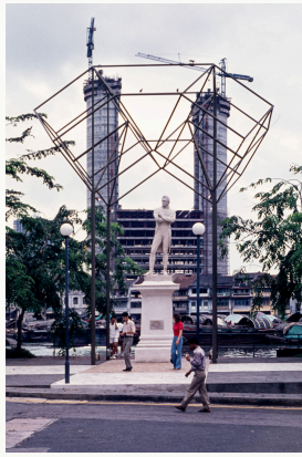
Raffle's Landing Site and the Construction of the OCBC-Building
