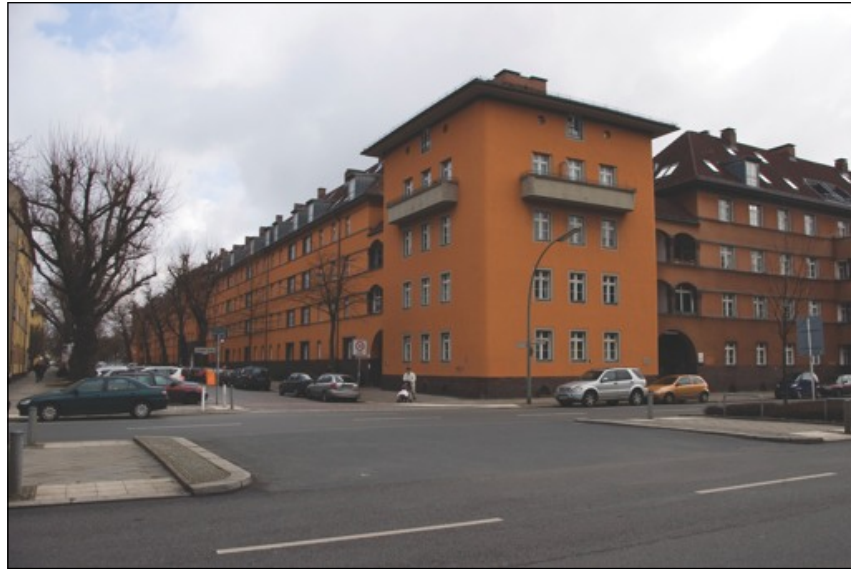
Figure 65: Corner, Anrumer- and Ostender Strasse. Author's own photograph.
