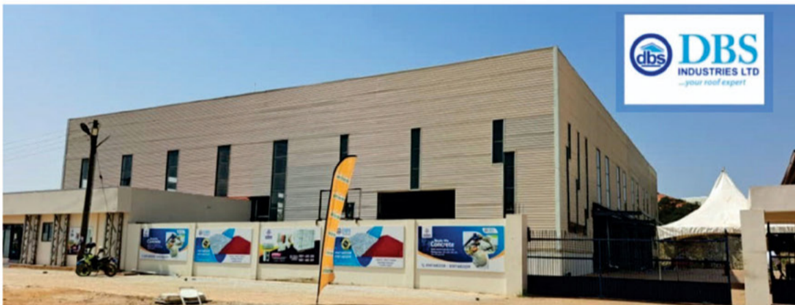
Factory building view
