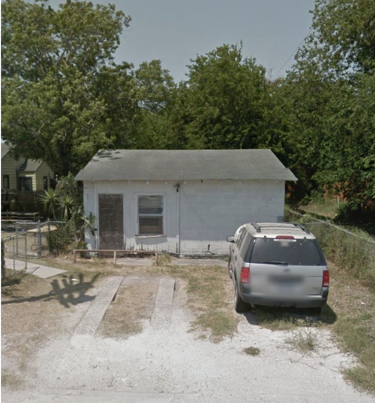
Potential Blight #5: Home in need of maintenance on E 4th St
