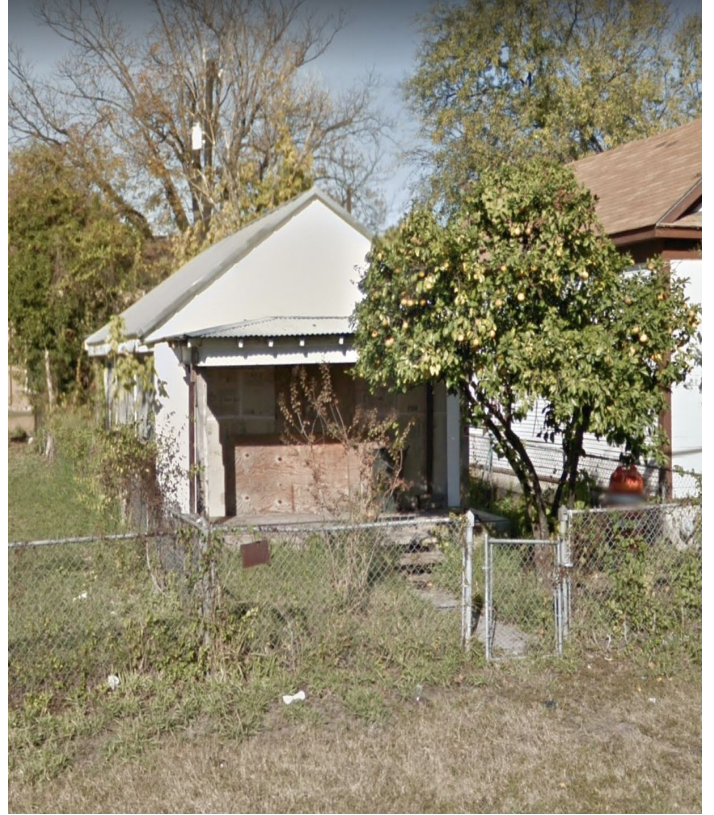
Potential Blight #2: Vacant Home on El Paso St.
