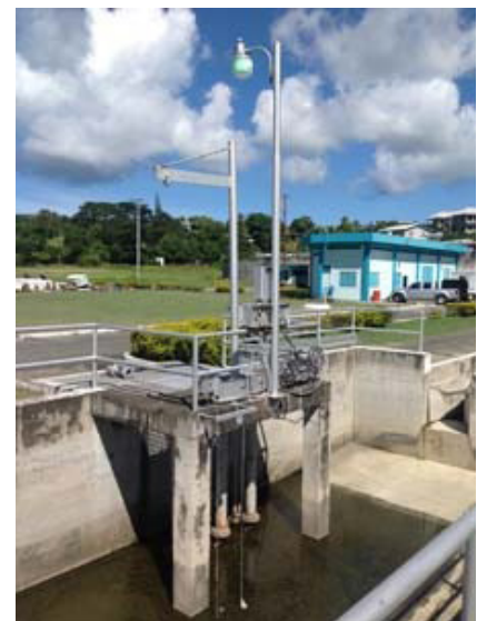
Water treatment plant in Scarborough, Trinidad Photo Credit: GEF-CREW
