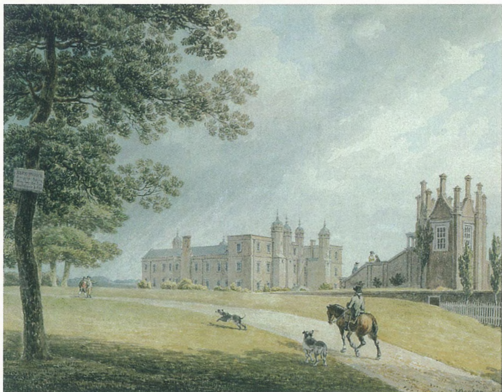
Plate VI. Melford Hall, watercolour by Michael Angelo Rooker, 1796. View at the entrance from Melford Green with the banqueting house on the right. The flat roof of the west wing can be seen clearly. The second-floor room of the north-west corner was the purple bed chamber in 1635. (By courtesy of Sir Richard Hyde Parker, Bt)
