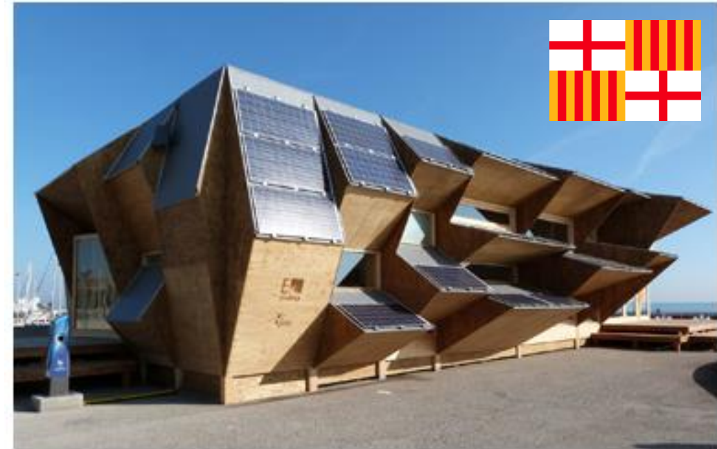
An innovative solar-powered building in Barcelona
