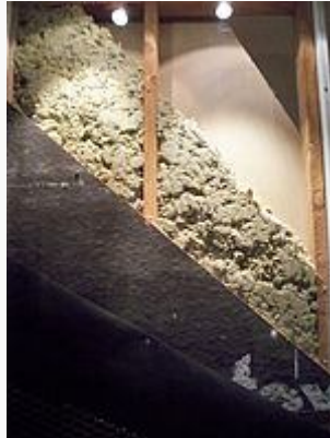
Cross-section of cellulose insulation
