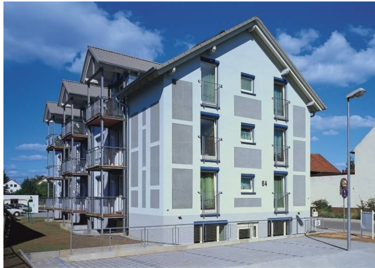
Transparent insulation Source: http://umwelt-wand.de
