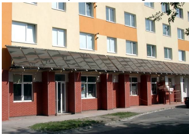
Solar collectors as a canopy Source: Sára Horvath
