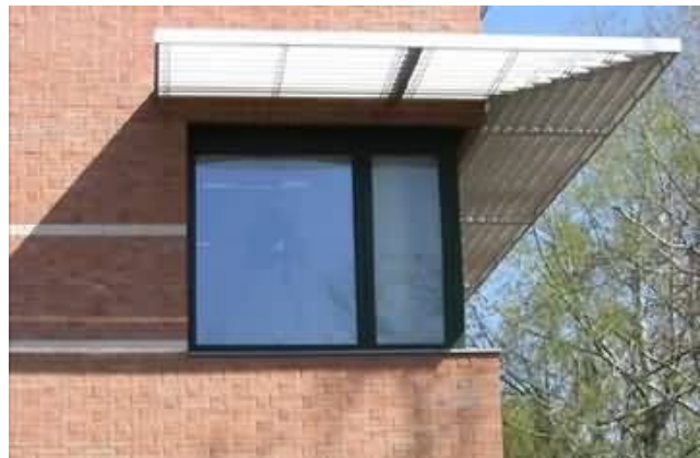
and fix horizontal louvers
