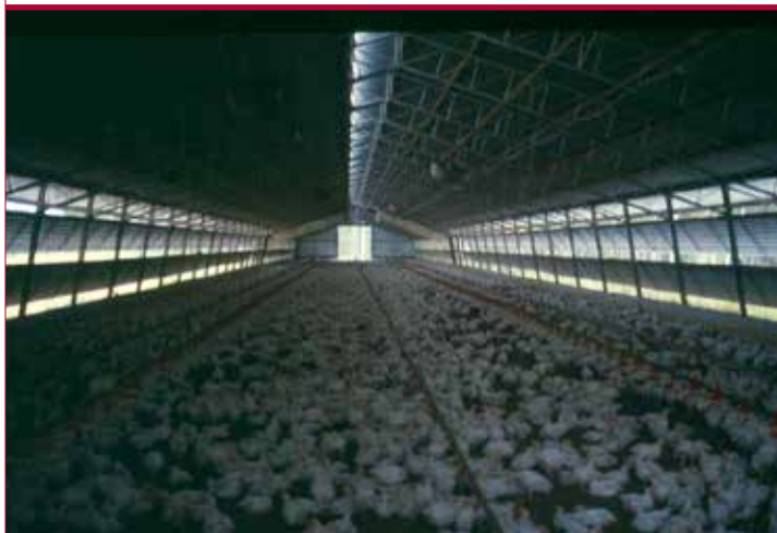
Large-scale naturally ventilated broiler house
