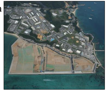
Construction of the Futenma Replacement Facility
