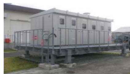
Elevation of Substation Facilities (Measures for Tsunami)
