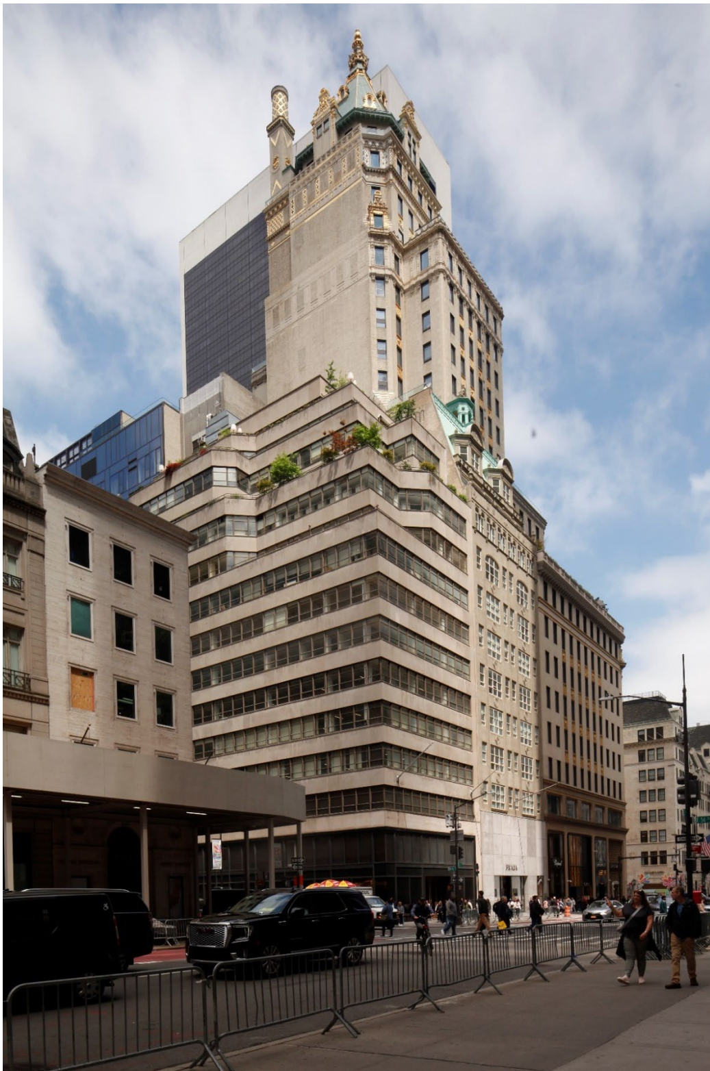
Heckscher Building, view from Fifth Avenue, south of 56th Street Sarah Eccles and Bilge Kose, May 2024
