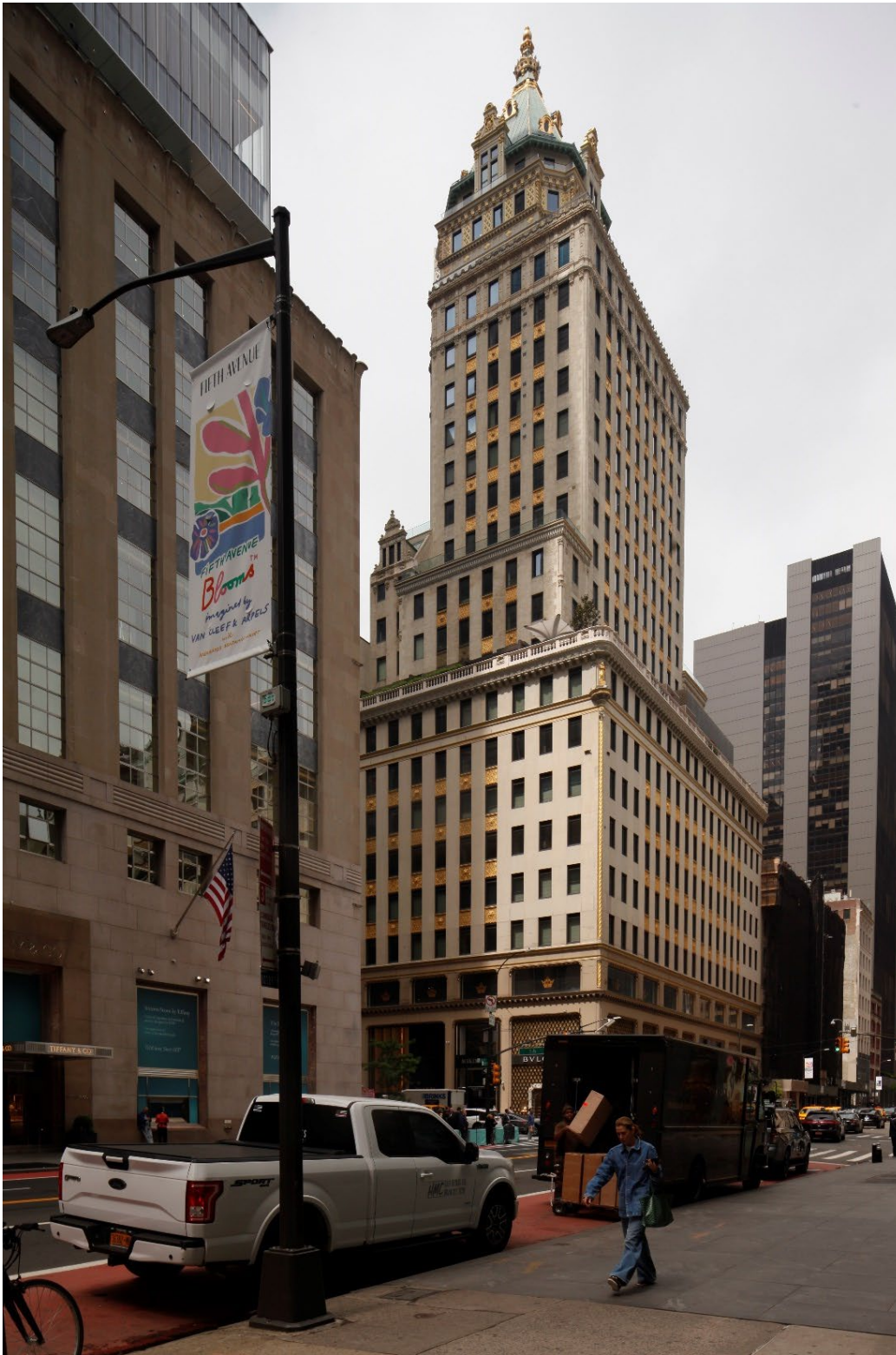
Heckscher Building, view from East 57th Street Sarah Eccles and Bilge Kose, May 2024
