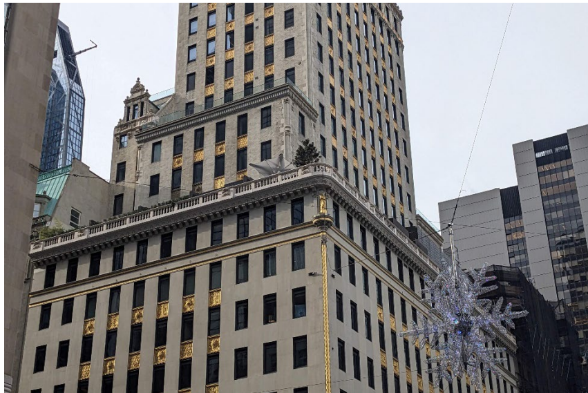
Corner, view from East 57th Street LPC, 2023
