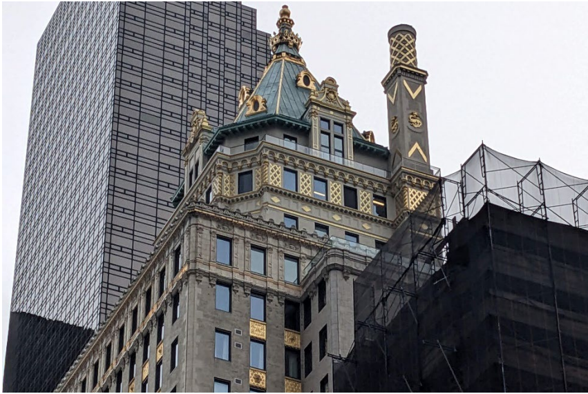
Crown, view from West 57th Street LPC, 2023
