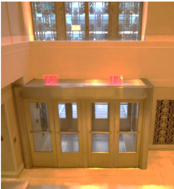
Park Avenue Foyer Side Vestibule
