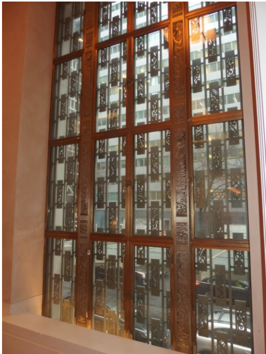
Park Avenue Window Detail
