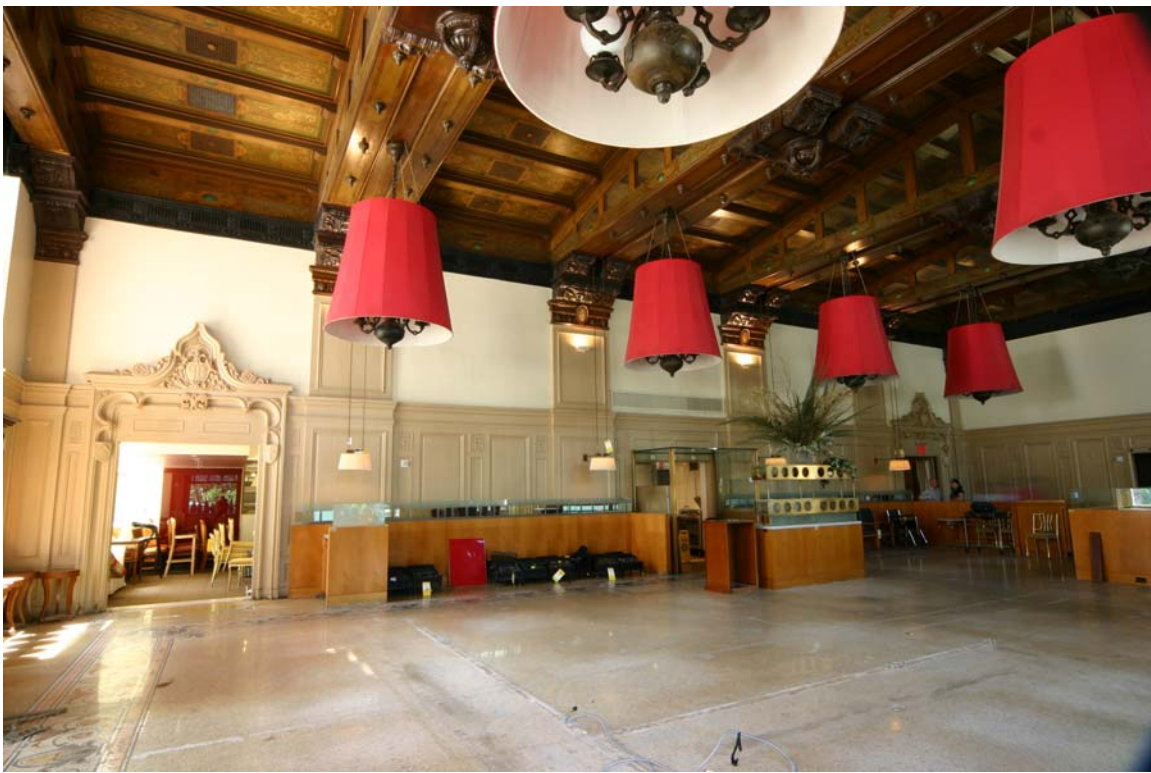
The Edwardian Room Ceiling and view south
