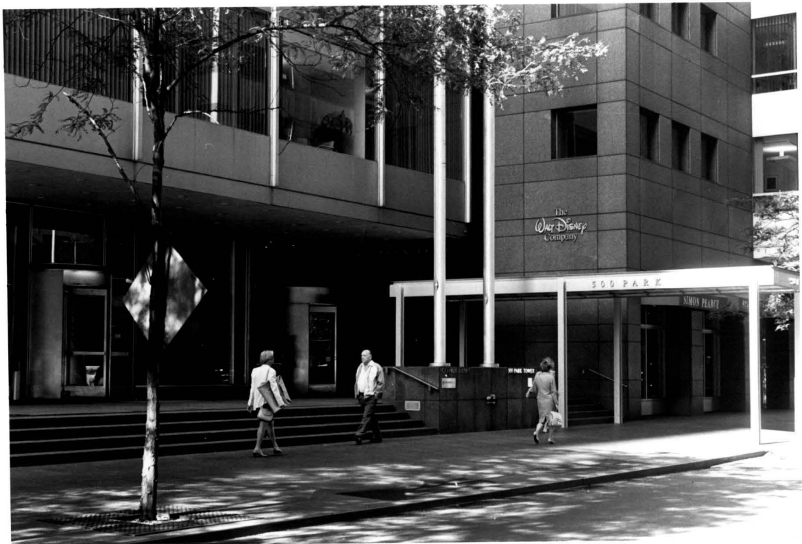
Fig. 8: detail of first story, Park Avenue facade (DMB) Fig. 9: view of first story, East 59th St. facade (DMB)
