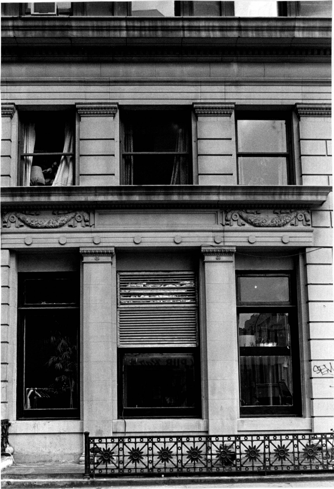
The Bank of the Metropolis 16th Street elevation, two-story base, detail
