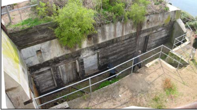
Figure C-6. 33: Engine house entrance, South Channel Fort (c1888).
