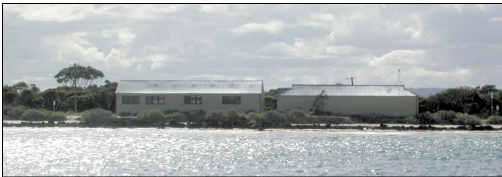
Figure C-6. 51: Swan Pt mine assembly sheds.
