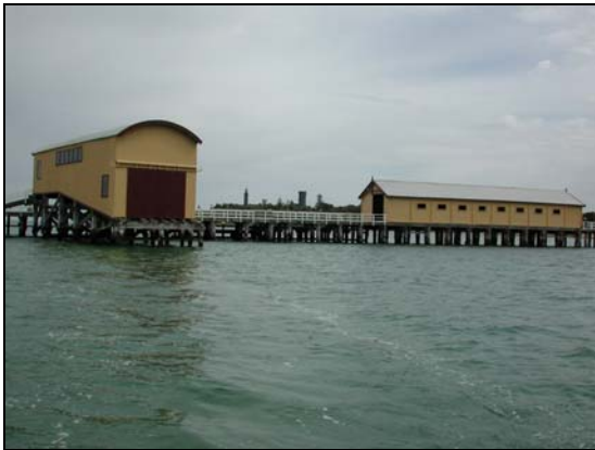
Figure D-1. 14: The Waiting Shed (right) on the New Pier.
