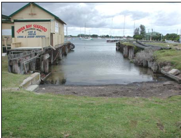
Figure E-9. 1: Locke's/Cayzers Brother's boat shed dock/ slipway.
