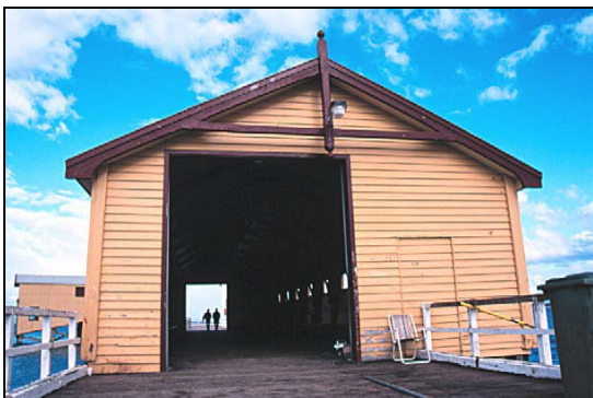
Figure D-1. 16: Queenscliff New Pier Waiting Shed, 2001 (Photo: M Gibbs).
