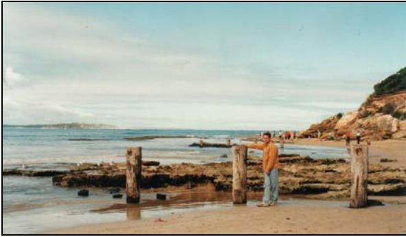
Figure D-1. 22: Pt Lonsdale sand groyne in 1994 prior to demolition.
