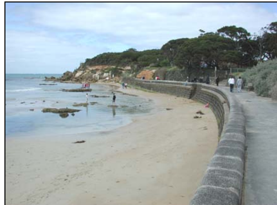
Figure D-1. 24: Pt Lonsdale seawall and promenade.
