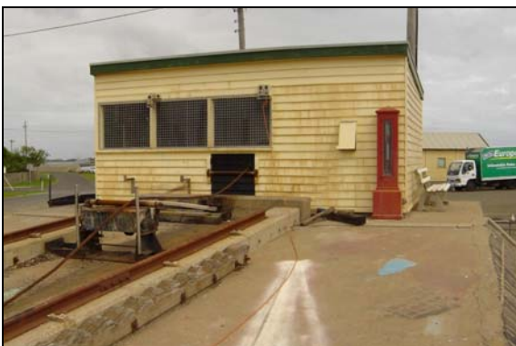
Figure E-9. 7: Queenscliff Slipway Winch Shed. Note former Fisherman's Pier Barometer and Fishermen's Meeting Place Seat on right.
