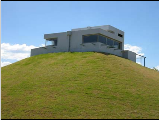
Figure C-6. 26: Fort Queenscliff dual DRF station, built 1915.
