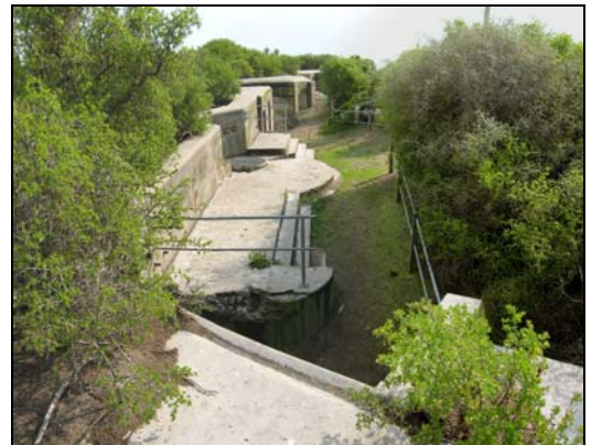
Figure C-6. 4: South Channel Fort.
