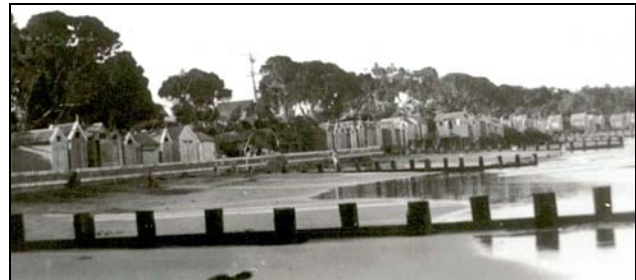
Figure D-1. 9: Pt Lonsdale Front Beach c. 1950s. Note the seawall built to protect the bathing boxes, and sand groynes (PH 3791, QHM Collection).
