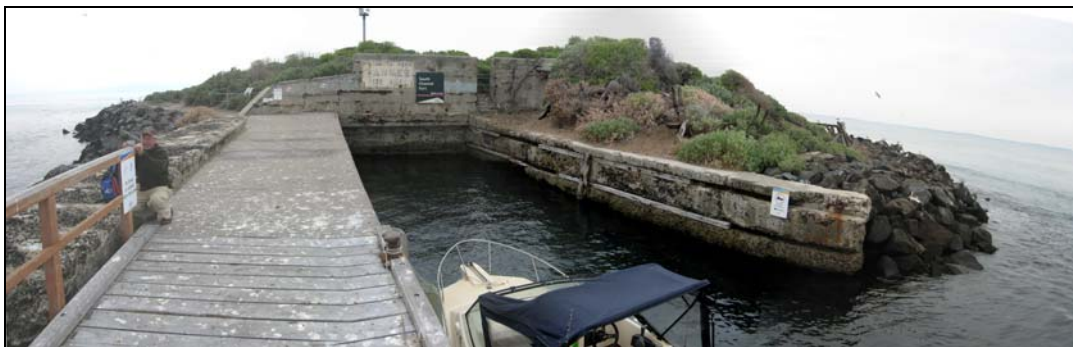
Figure C-6. 79: South Channel Fort Dock for torpedo boats.
