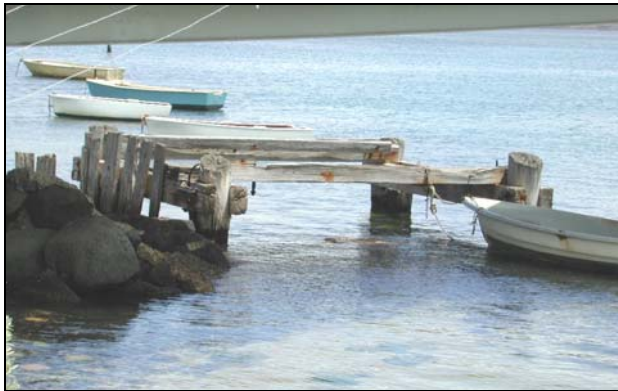
Figure C-6. 77: Old Swan Island Bridge.
