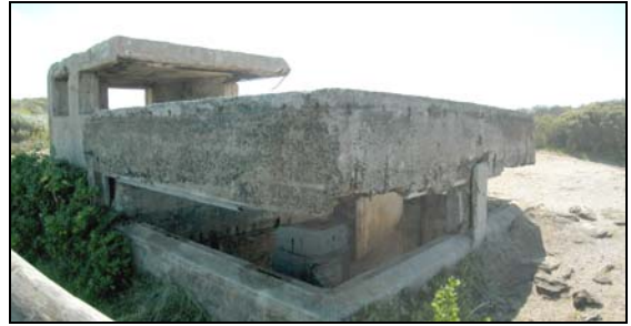
Figure C-6. 22: Pt Lonsdale WWII DRF Station. Note that the top structure (on right) was formerly an electric (search) light detector (E.L.D.).
