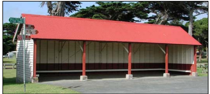
Figure D-1. 15: Waiting Shed near New Pier.
