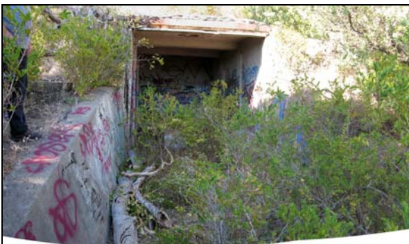
Figure C-6. 35: Pt Lonsdale WWII generator shed bunker (c. 1942).
