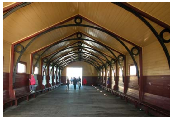
Figure D-1. 17: Interior of Queenscliff New Pier Waiting Shed.
