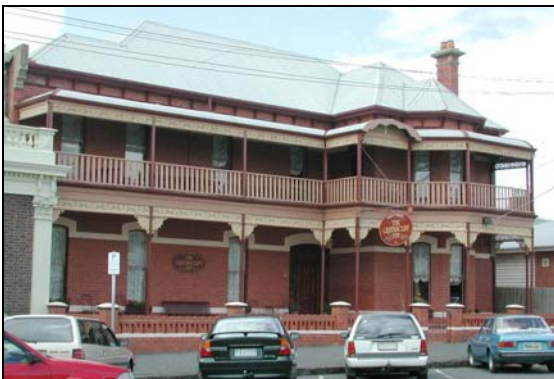
Figure D-1. 33: Queenscliff Inn.
