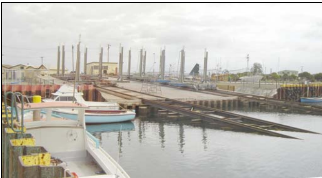
Figure E-9. 6: Queenscliff Slipway.
