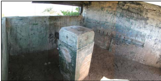
Figure C-6. 18: Pt Lonsdale DRF station interior, showing alidade pedestal mounting.
