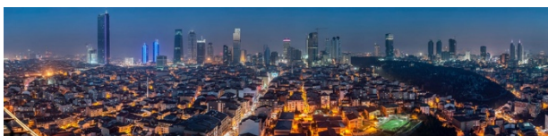
Figure 1 & 2: Istanbul business district from an airplane (up), from a skyscraper (down). Photos: M. Germen.
