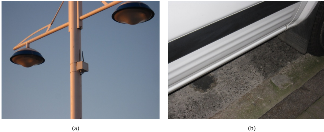
Figure 4. (a) Wireless sensor nodes attached to lamppost; (b) Wireless sensor nodes buried under the asphalt
