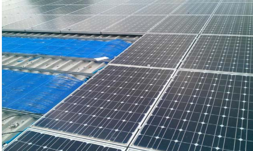
Figure 2. PVT/water system (appropriate for BI applications) studied by Buker et al. [61]: a) the heat exchanger loop underneath the PV modules, b) the thermal roof unit piping and c) the prototype of the proposed system (Source: [61]).
