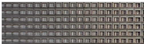
Figure 8. Morphing of house textures by linearly interpolating between two different textures. The disentangling properties of PSGAN allows to morph in a controlled manner: the house window periodicity stays the same, but the facade type and appearance change significantly due to the changing global dimensions.
