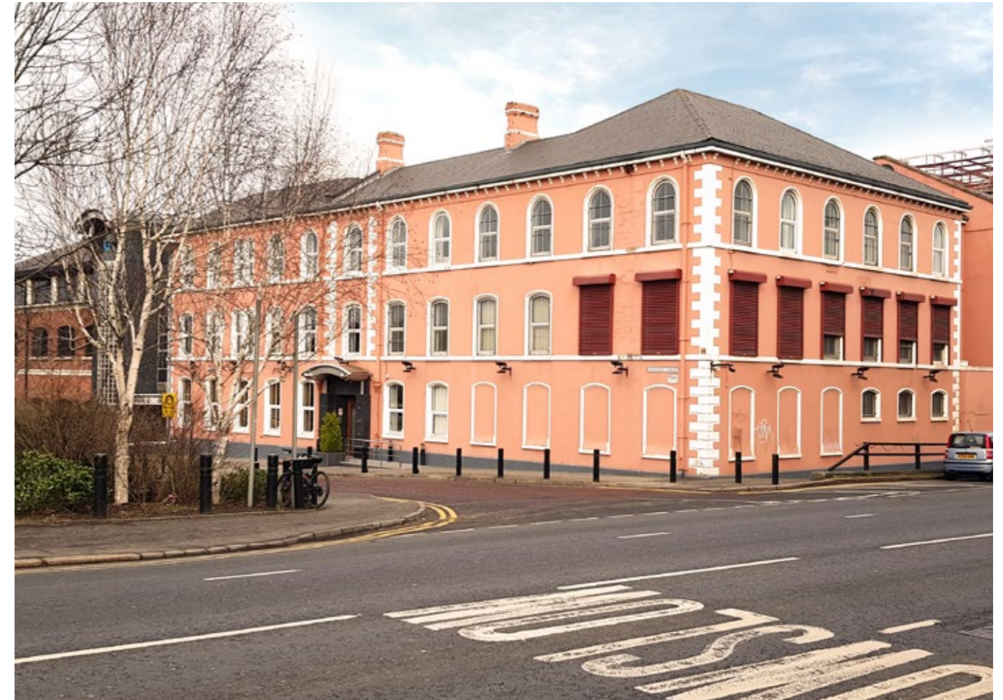
CONSULTANCY &amp; DISPOSAL - CASE STUDY
