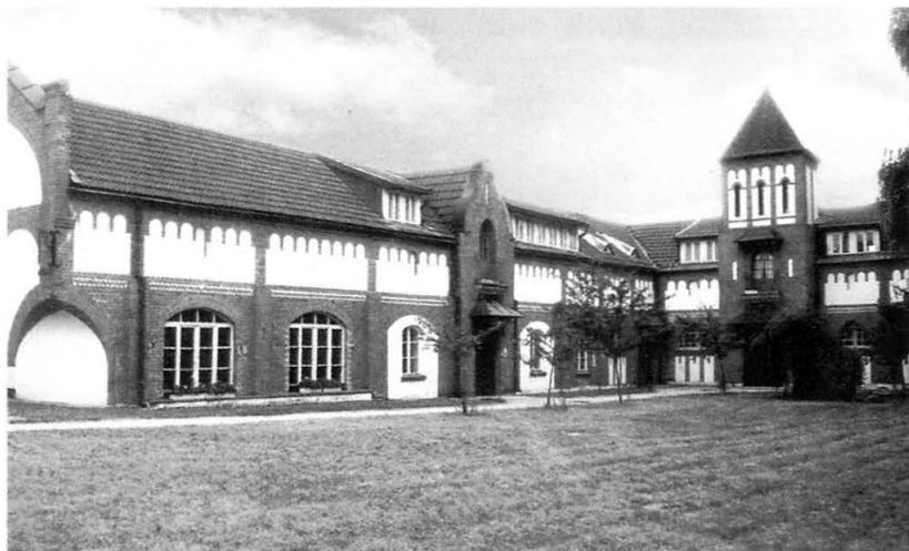
20. Budynek stajni i wozowni. Stable and coach house.
