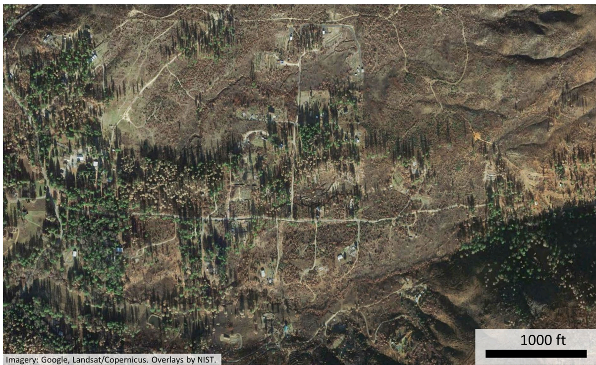
Figure 6. WUI Type 6: Low Density Intermix: Concow, CA. Note the overall large SSD and structures located within the wildland vegetation. Note the imagery is taken after the 2018 Camp Fire.
