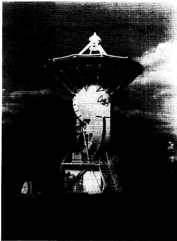
A 30-ft Apollo Unified S-Band System antenna and operating console at Goddard's Network Test and Training Facility at Goddard Space Flight Center.
