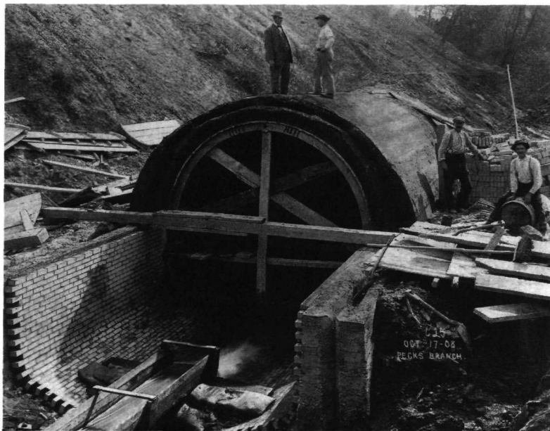
Construction of a storm drain at Pecks Branch. Photograph by Alfred Waldeck, 1908. (Courtesy Baltimore Public Works Museum.)
