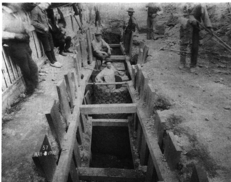
Bracing and manhole construction for storm drains and sewers. Photograph by Alfred Waldeck, 1907. (Courtesy Baltimore Public Works Museum.)
