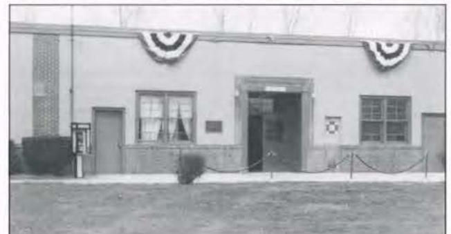
DECKED OUT: A Gill area building at Montrose, site of the Maryland Military Academy, readied for guests. (Photo by Sgt. Ed Billips)
