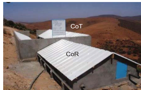
Figure 3: Two slopes roof condenser (CoR) and condenser on terrace (CoT).
