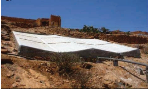
Figure 4: Condenser on ground CoG.
