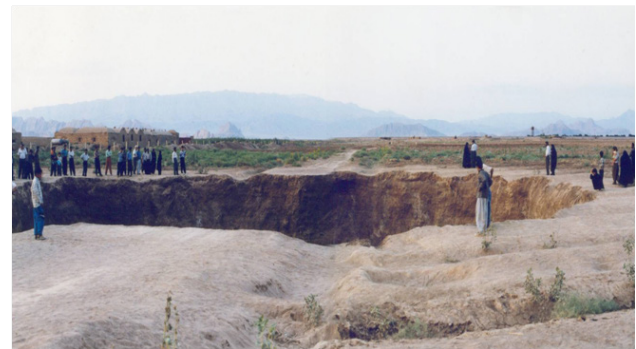
Figure 3 Land subsidence in Kerman region in Iran.
