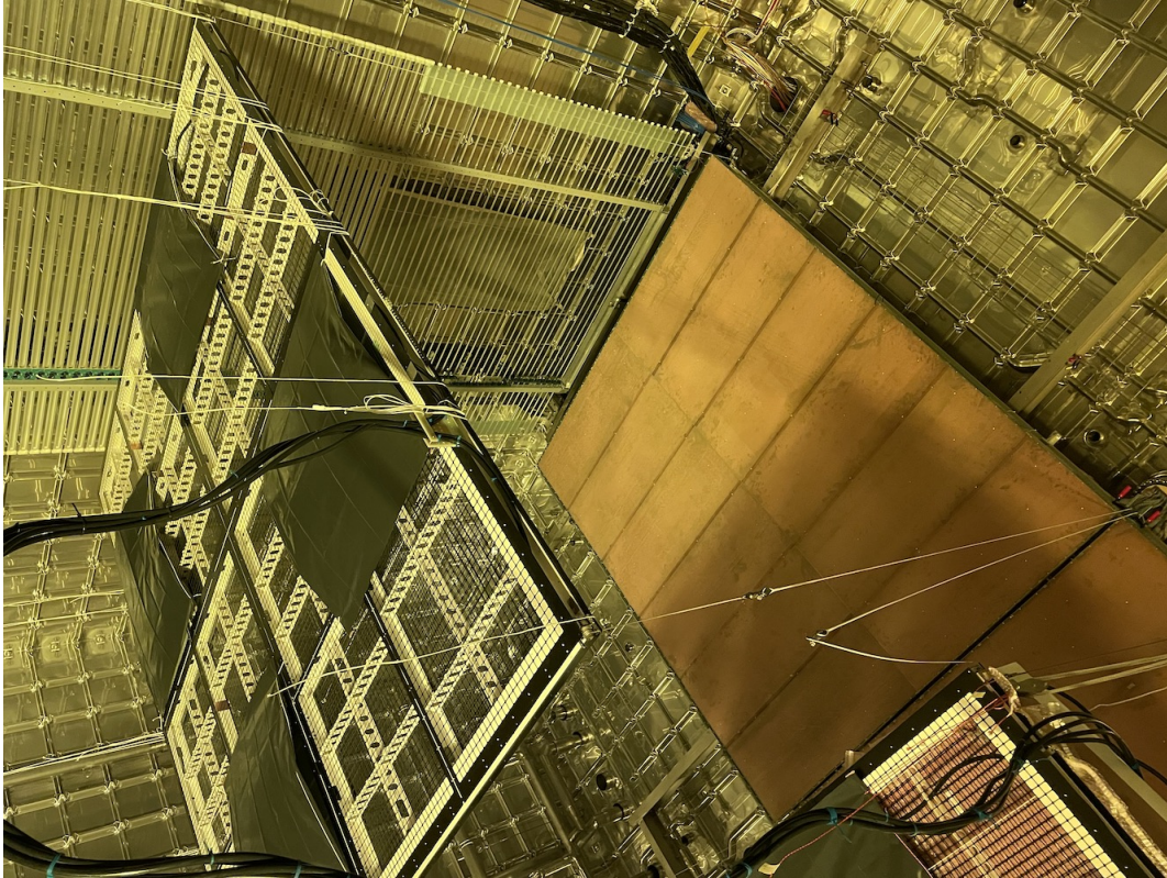
Figure 8.1: The inner volume of NP02 during installation of the FD2-VD Module 0 detector. The two top charge-readout planes (CRPs) are visible, along with one cathode equipped with four sensors, the downstream cathode is temporarily elevated and two X-ARAPUCAs on the upstream wall are visible behind the upstream field cage (the downstream membrane wall X-ARAPUCAs are not visible). All of the X-ARAPUCAs are covered by temporary bags.
