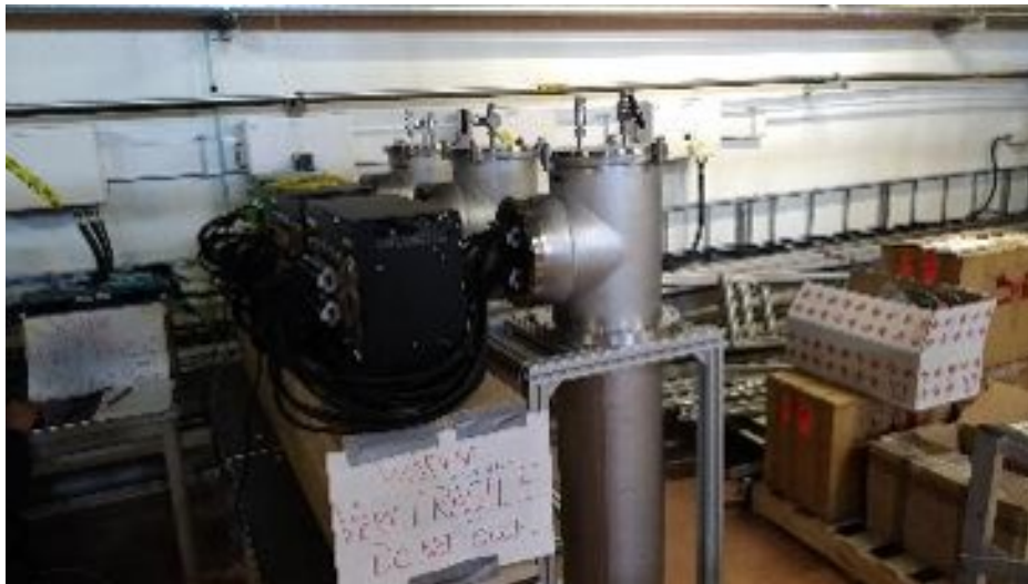
Figure 4.27: TDE integration test at EHN1 in summer 2021
