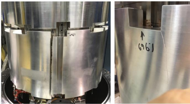
Fig. 8. (L) Fractured shell on the non-lead-end of MQXFAP2. (R) Initiation of a crack from the sharp corner of a different quadrant of the shell.
