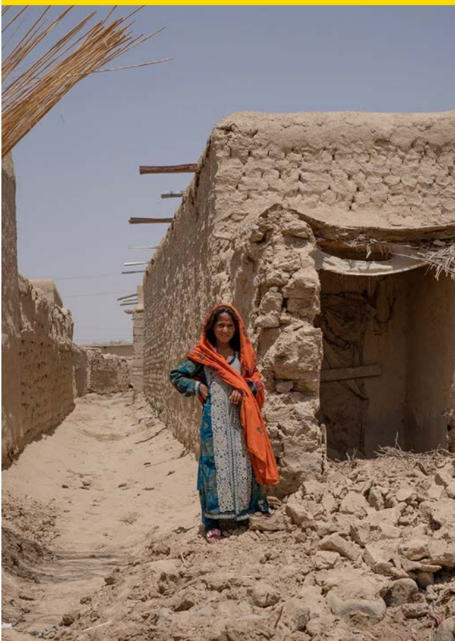
Figure 3. The condition of the housing of family3.
