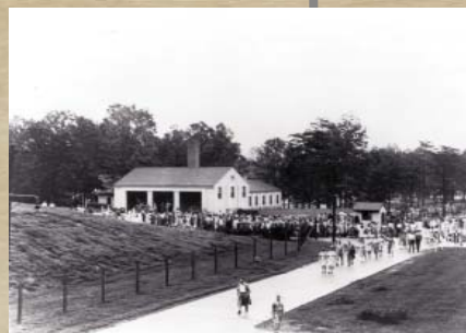
14 JUN. The Army assumed control of Arlington Hall, near Washington, DC. It would become the center of the Army's code-breaking and communications security efforts for the next five decades.
