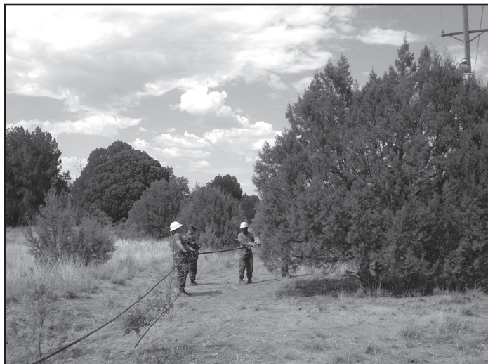
11 th Signal Brigade soldiers installing aerial fiber optics.
