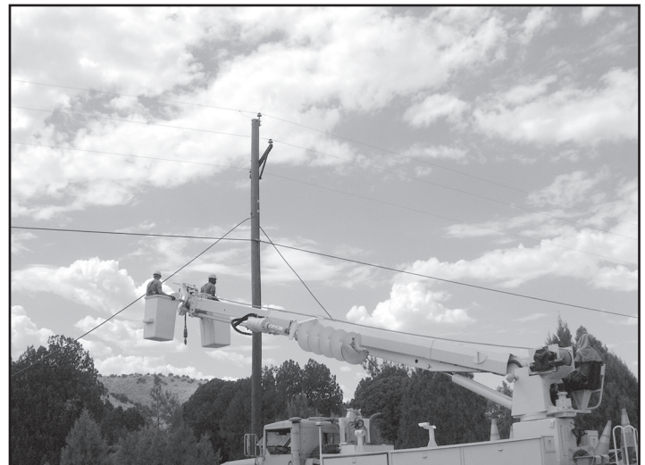
11 th Signal Brigade soldiers installing aerial fiber optics.
