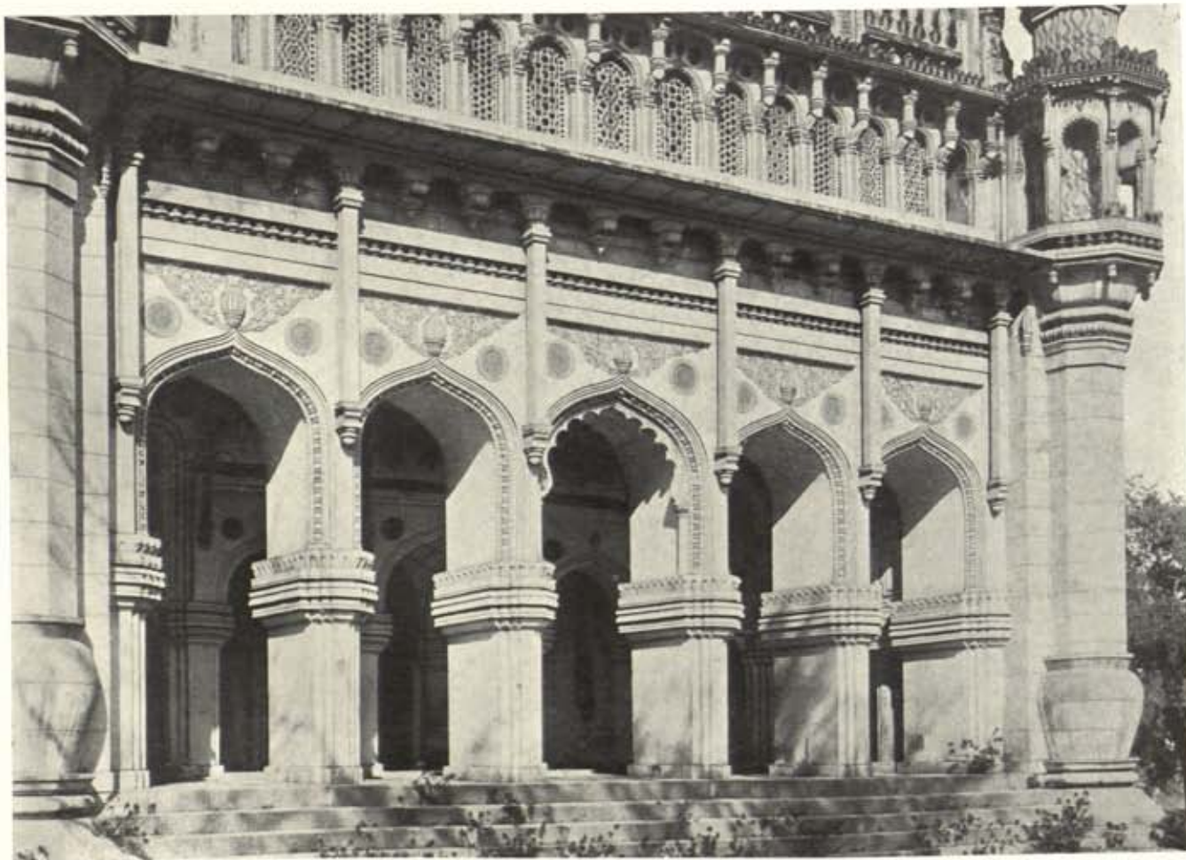
(c). THE SAME, COLONNADE, FRONT VIEW.
