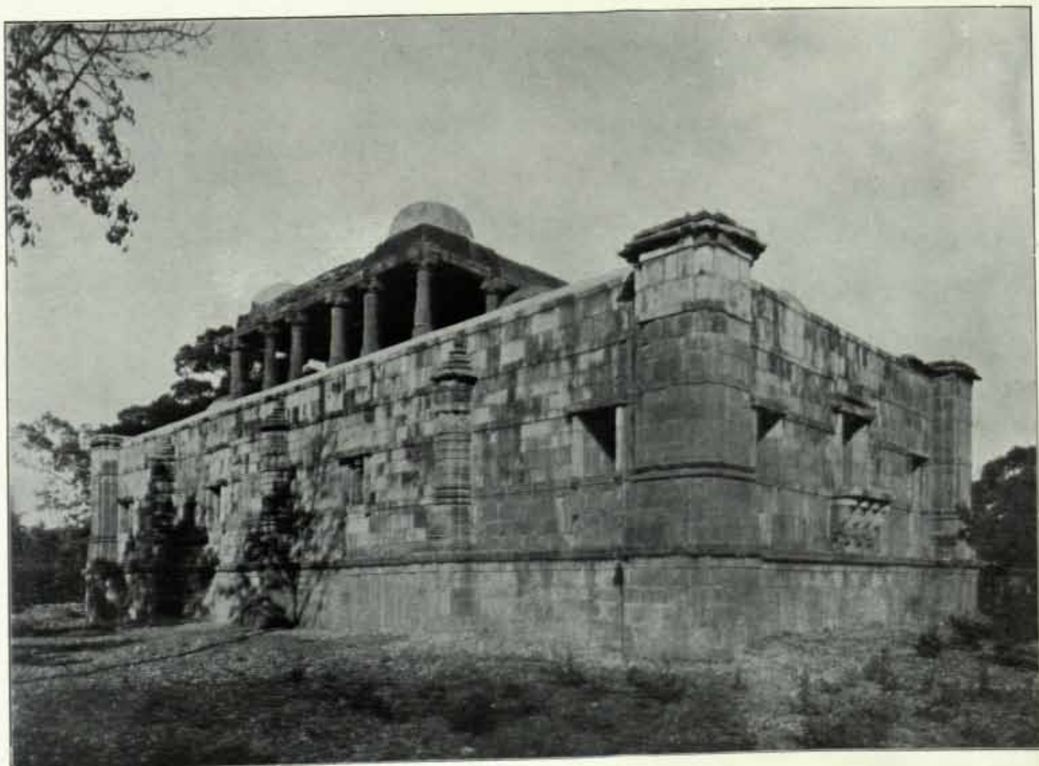
(b) NAGINA MASJID, CHAMPANER: AFTER REPAIR (BACK).
