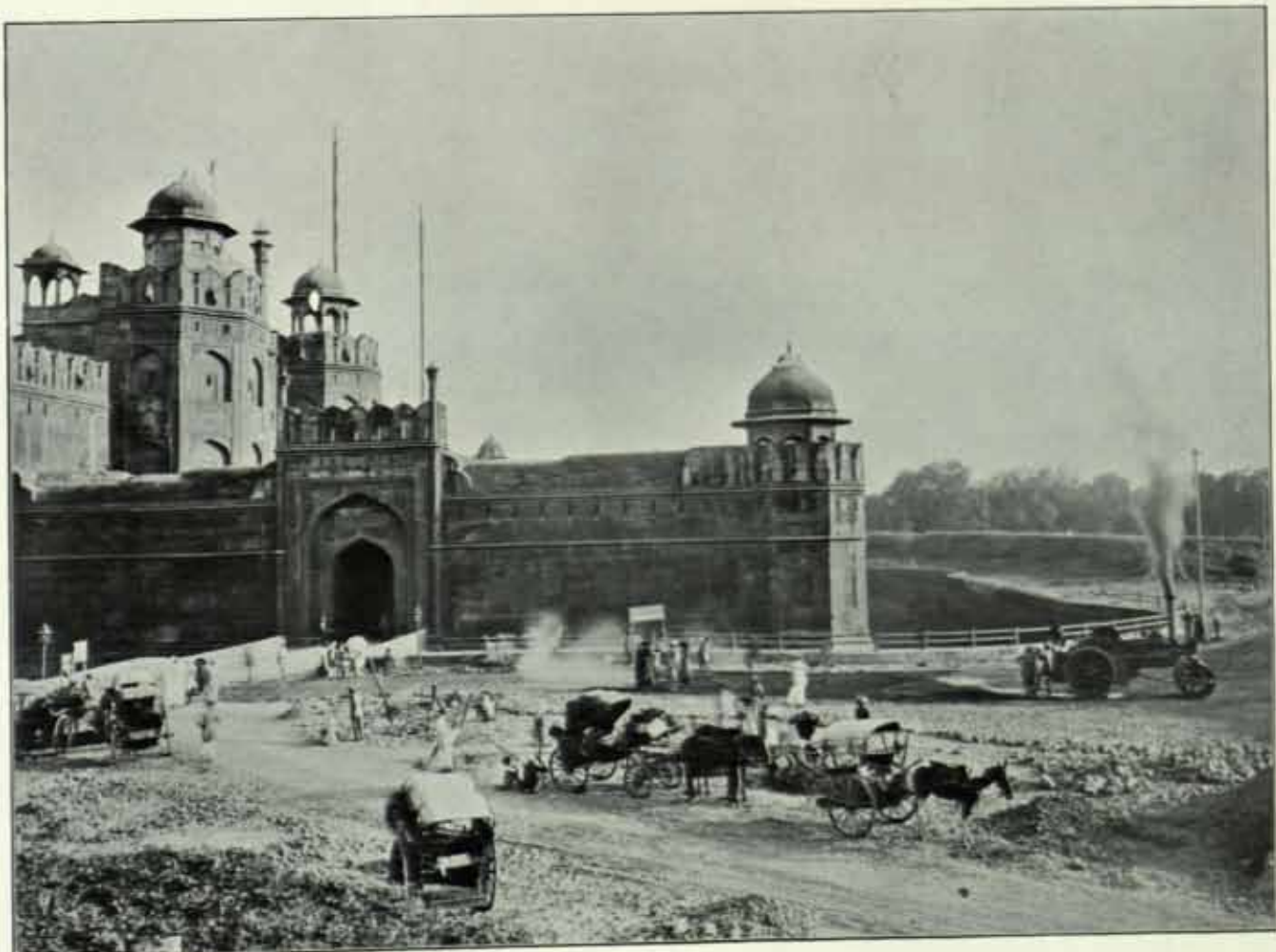
(b) LAHORI GATE, DELHI FORT: DURING REMOVAL OF EARTHWORK.
