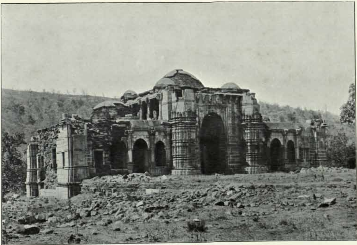
(a) NAGINA MASJID, CHAMPANER: BEFORE REPAIR (FRONT).
