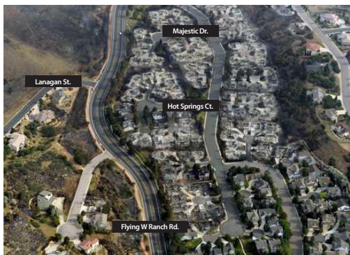
Figure 9: Majestic Drive area of the Mountain Shadows neighborhood after the Waldo Canyon Fire. Source: Colorado Springs Division of the Fire Marshal.
