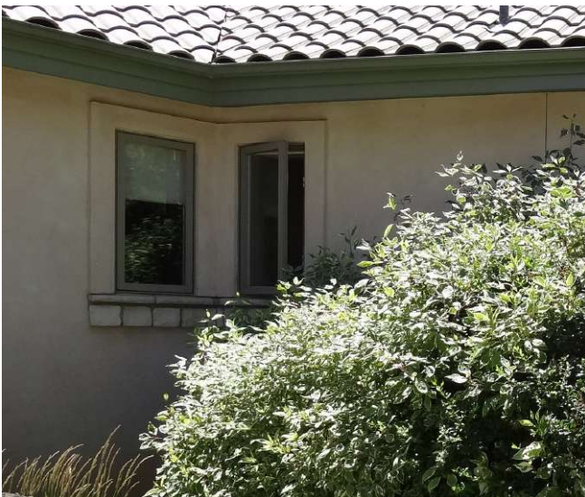
Figure D10: Near-home vegetation was prevalent at the front of this home. Note the open window in the lower photograph. Source: IBHS.
