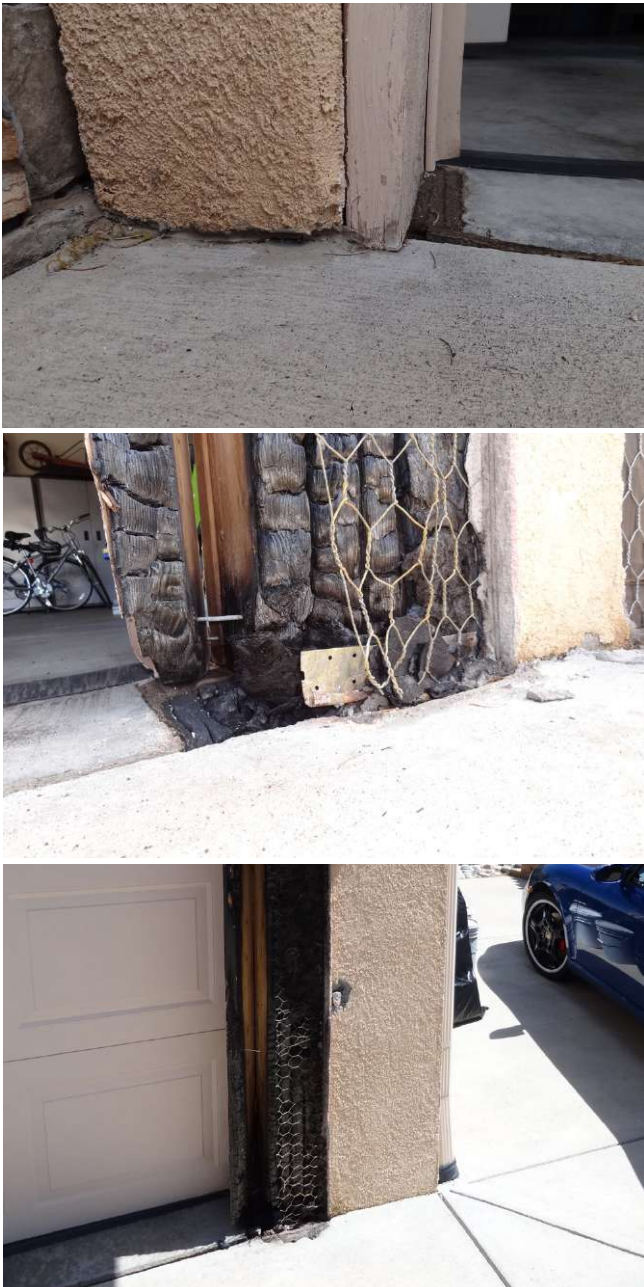
Figure 19: Photographs of the left, middle and right side columns of the two-car garage at a home on Lanagan Street. Note the low clearance between the concrete driveway and the EIFS system, as shown in the left-hand side column. The metal weep screed is visible at the base of the middle column. Source: IBHS.
