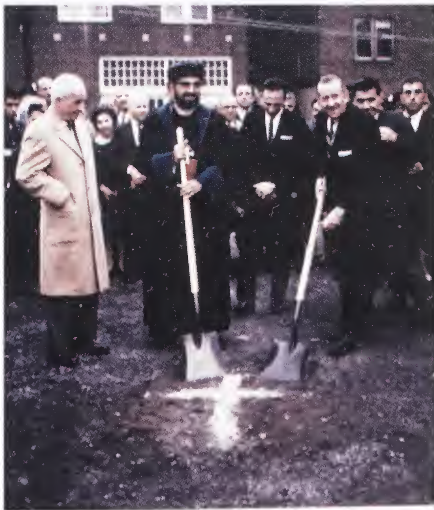
20. Ground breaking for the Mar Mari Slecha Church in Yonkers, New York in January 1967.
