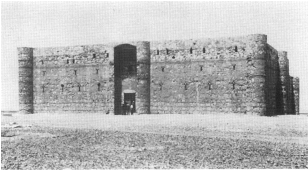
a. General view, showing the main entrance with quarter-round towers (upper section restored)
